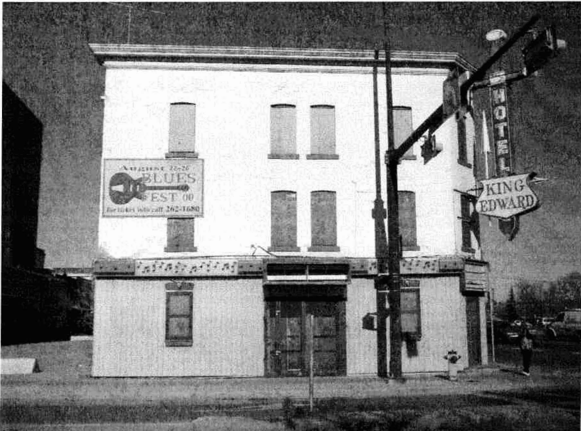
(Photo #1.1: The South Façade of the King Edward Hotel)
