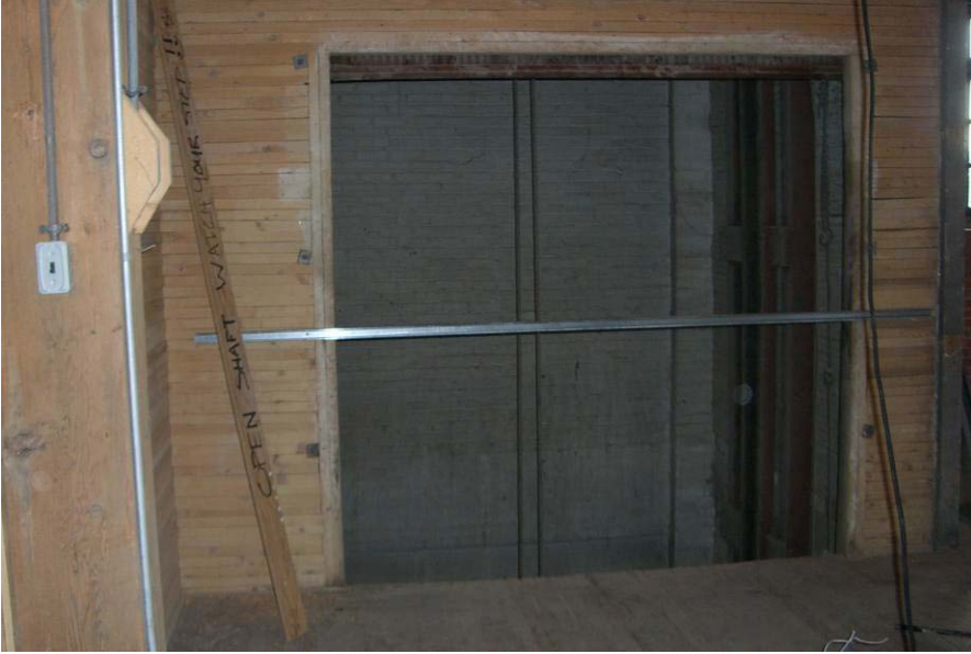
(Photo # 5. 4: The freight elevator shaft and its wood-frame enclosure)
