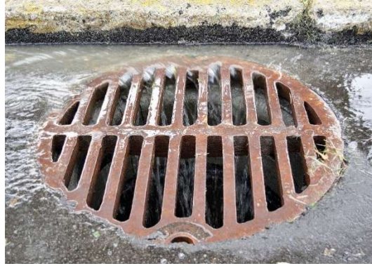
Figure 3.2: Flat Catchbasin Grate 1
