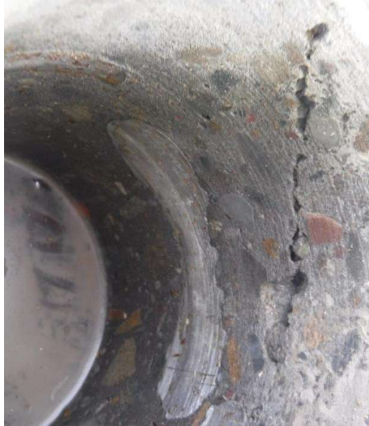
Figure 3.7 Cracked Manhole 6
