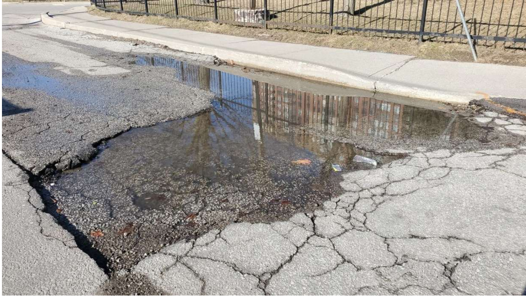
Figure 3.10 Surface Settling 9
