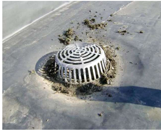
Figure 3.12 Roof Drain 10
