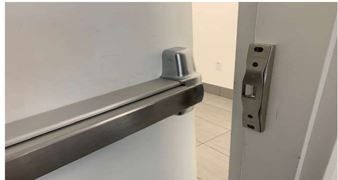
Strike plate allowing the door to mechanically override the lock
