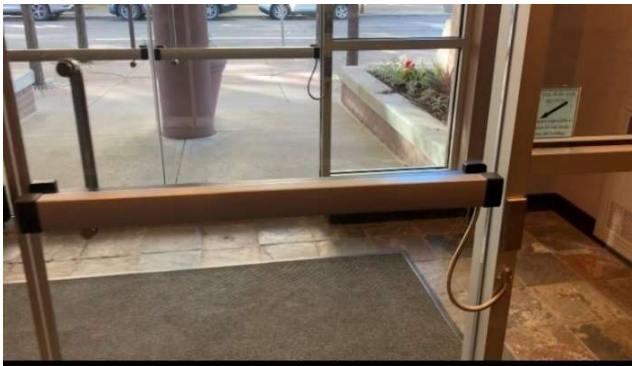
Figure 2: Panic hardware tied into the magnetic lock
