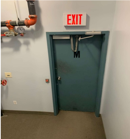
Figure 1: The images portray “push to exit” buttons. These require special knowledge, are not door hardware, and require two motions to open the doors.
