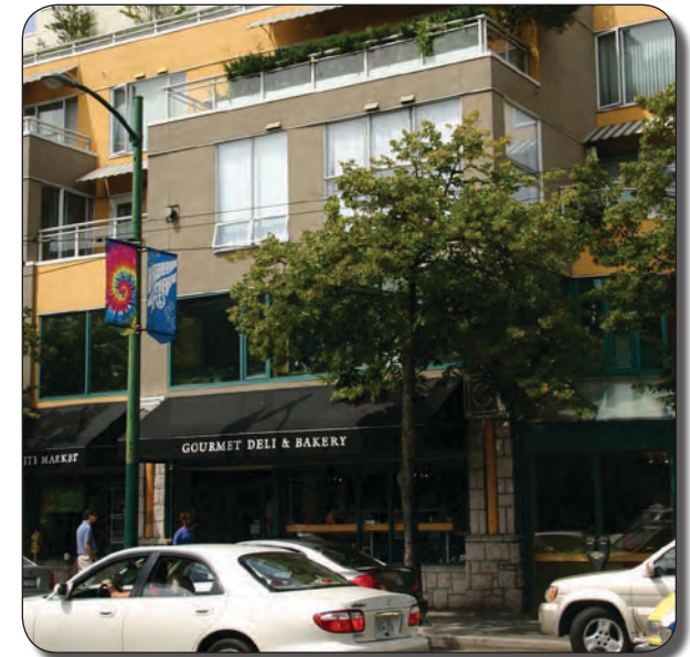
Canopies and awnings add to the visual interest and provide weather protection
