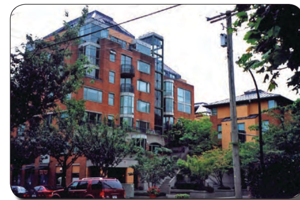
Medium density mixed use building
