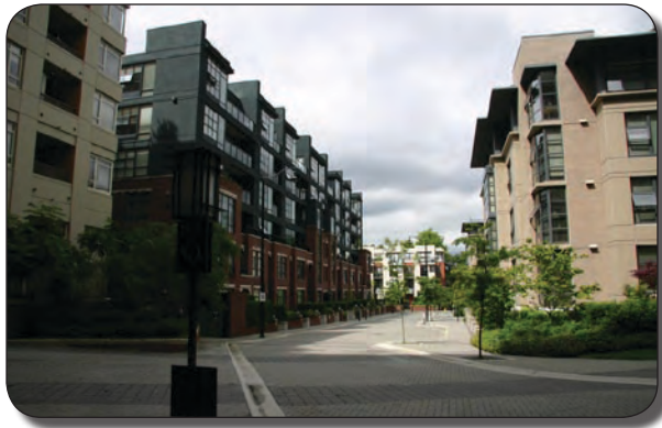
4 to 5 storey residential buildings
