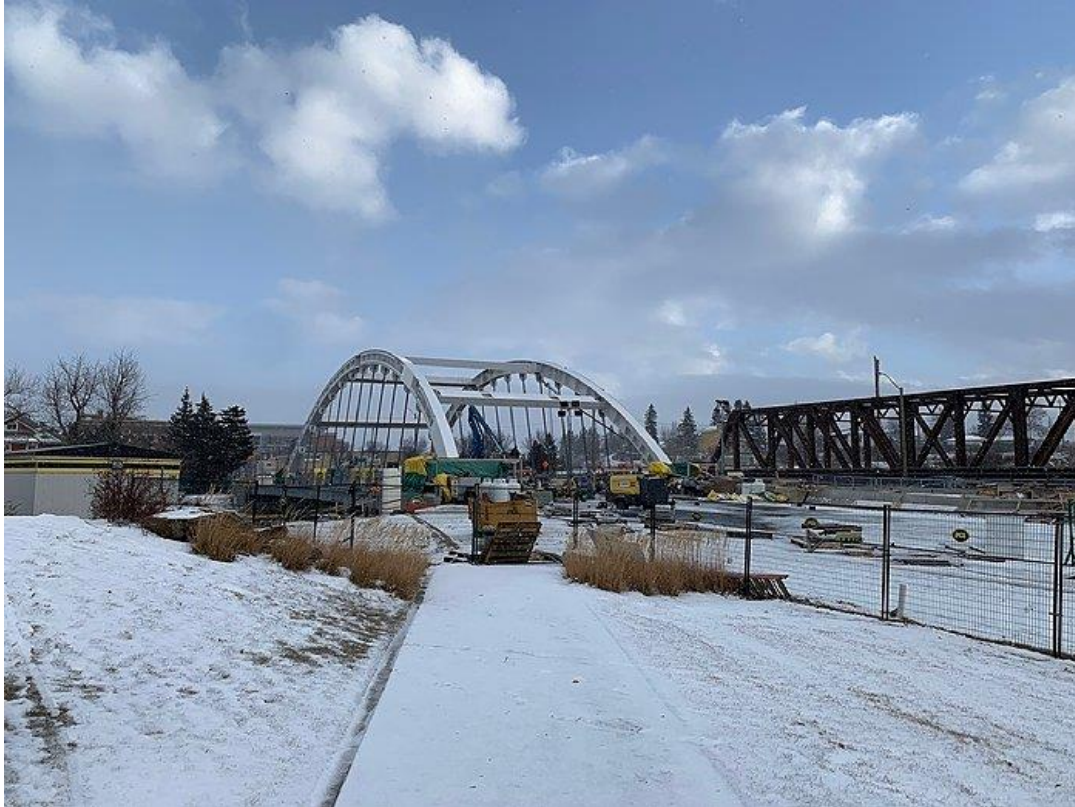
Progress on the 9 Avenue S.E. bridge.
