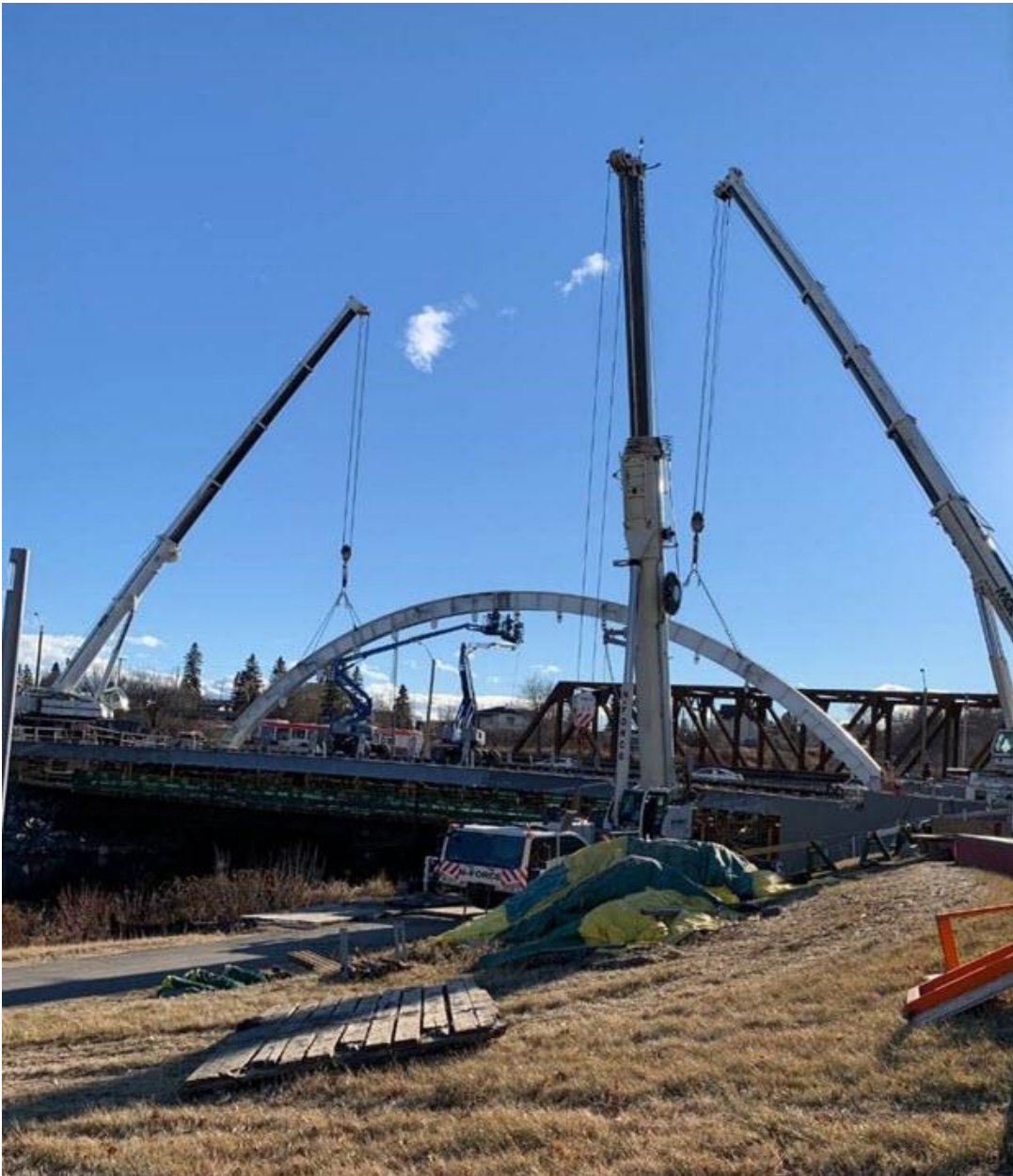
The first arch being installed on the bridge.
