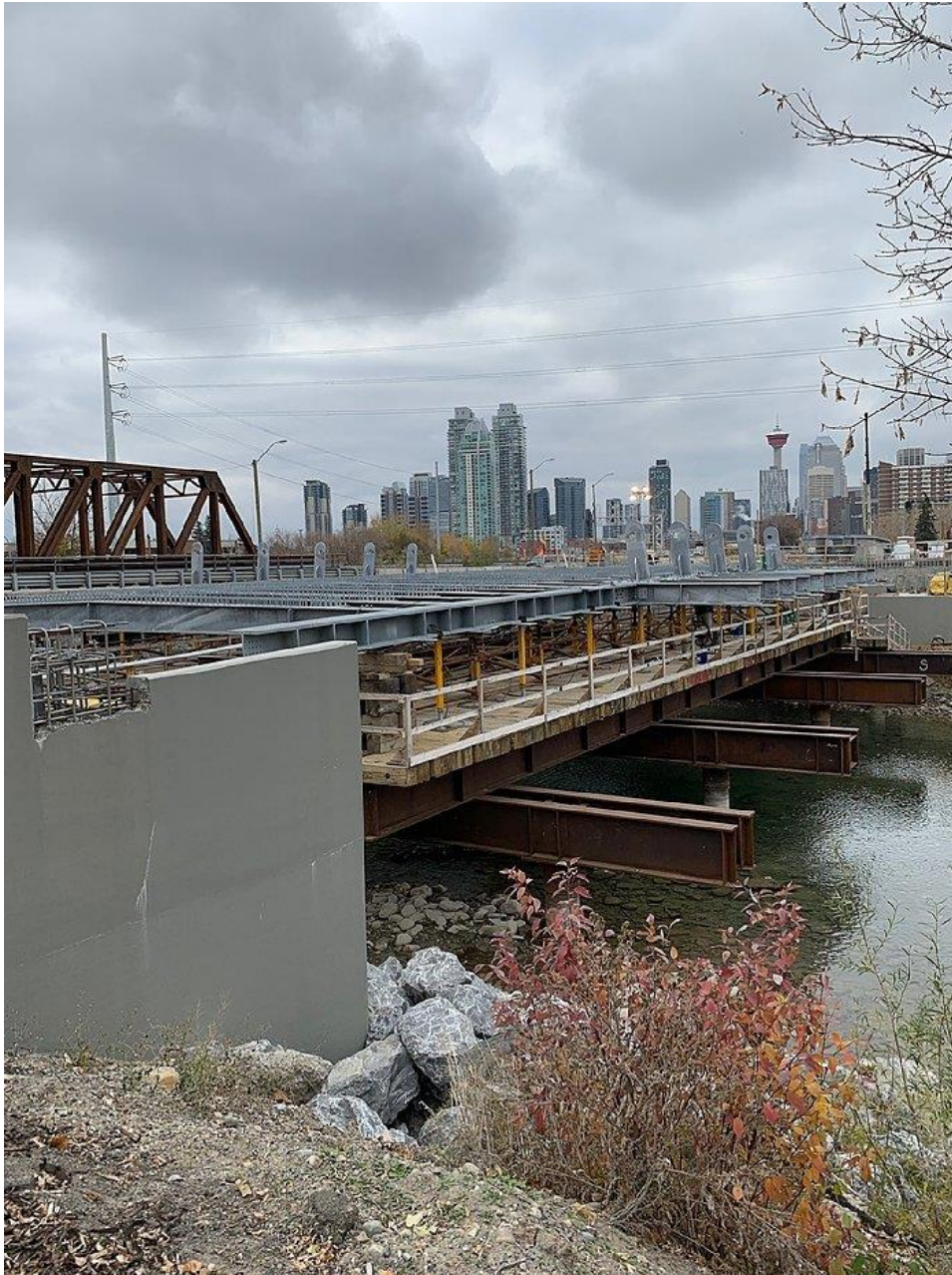
Progress on steel installation for the 9 Avenue S.E. bridge.
