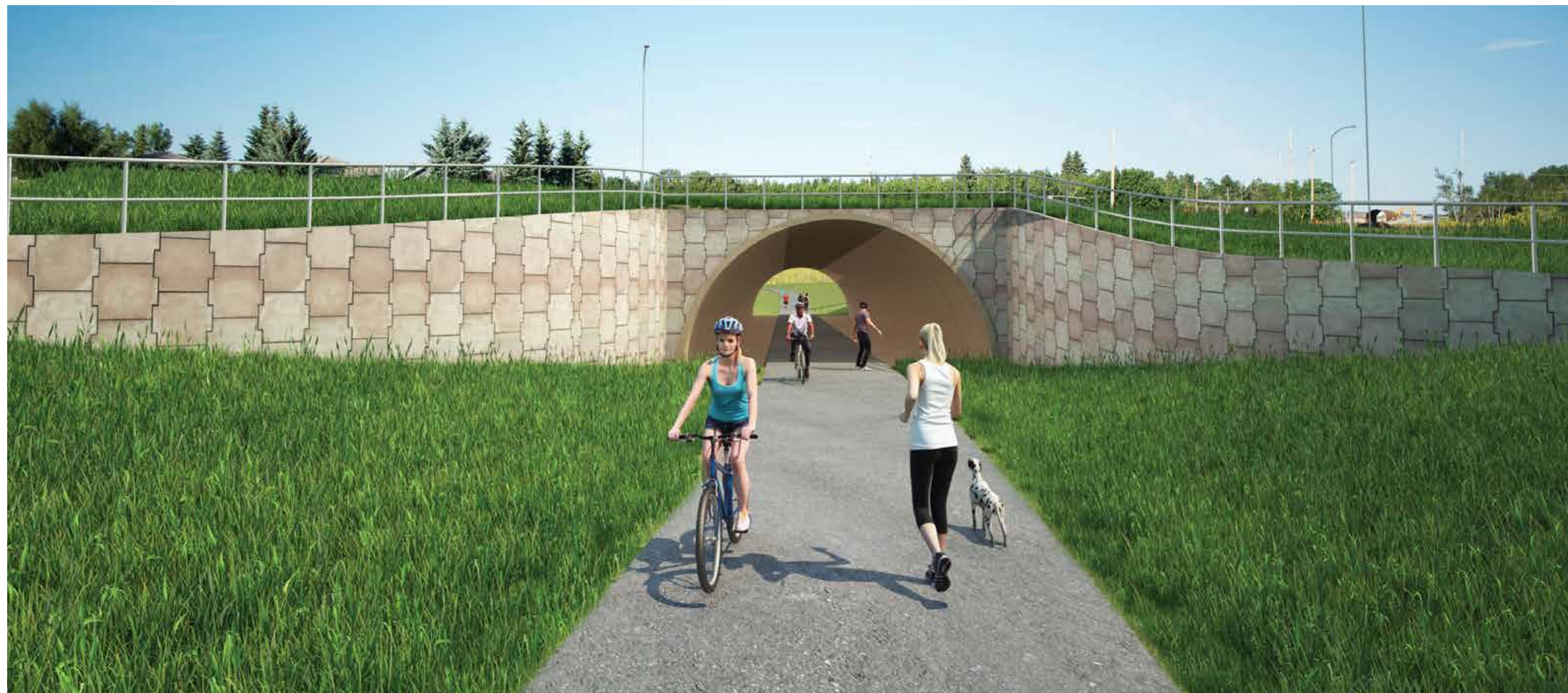
90th Ave. S.W. Approaching underpass from the north
