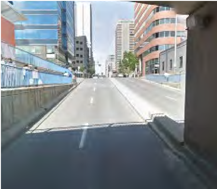
09 9TH AVENUE BRIDGE STRUCTURE - 8TH STREET
