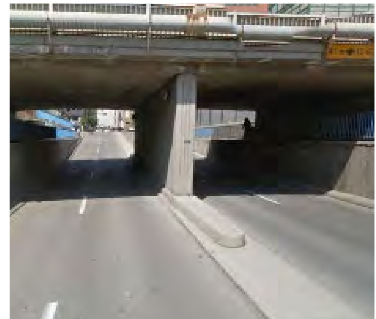
07 9TH AVENUE BRIDGE STRUCTURE - 8TH STREET
