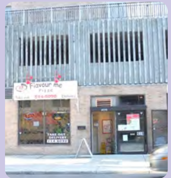
POOR COMMERCIAL FRONTAGE @ 8TH ST AND 5TH AVE
