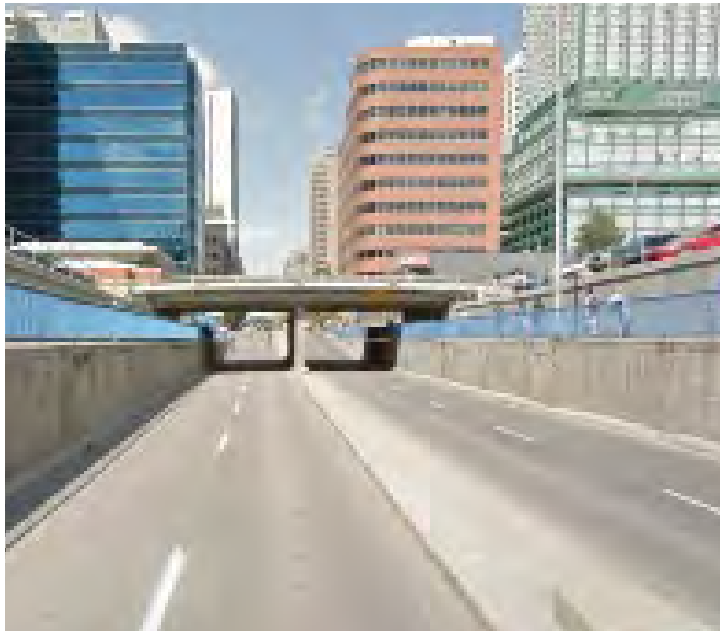
05 9TH AVENUE BRIDGE - 8TH STREET
