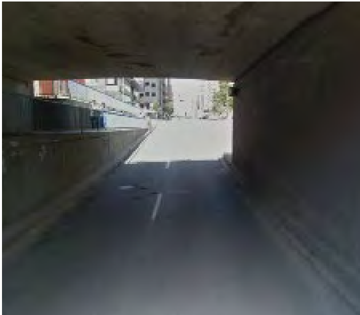
08 9TH AVENUE BRIDGE STRUCTURE - 8TH STREET
