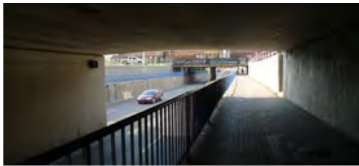
04 HARSH PEDESTRIAN UNDERPASS ENVIRONMENT.
