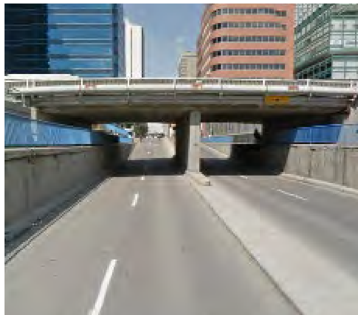
06 9TH AVENUE BRIDGE - 8TH STREET
