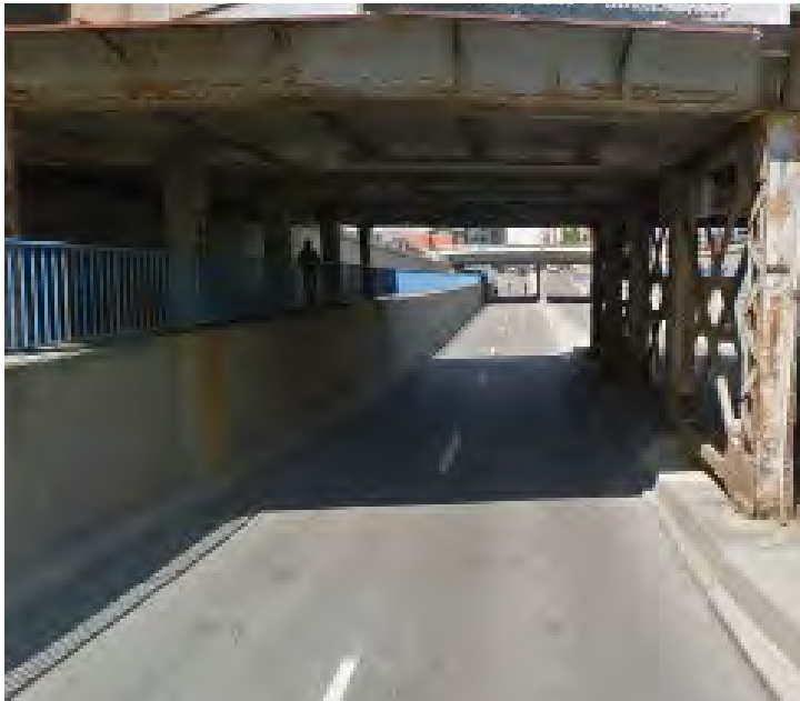
03 CPR BRIDGE STRUCTURE - 8TH STREET
