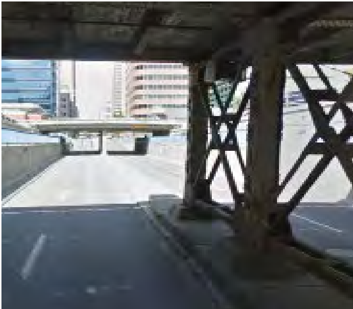
04 CPR BRIDGE STRUCTURE - 8TH STREET
