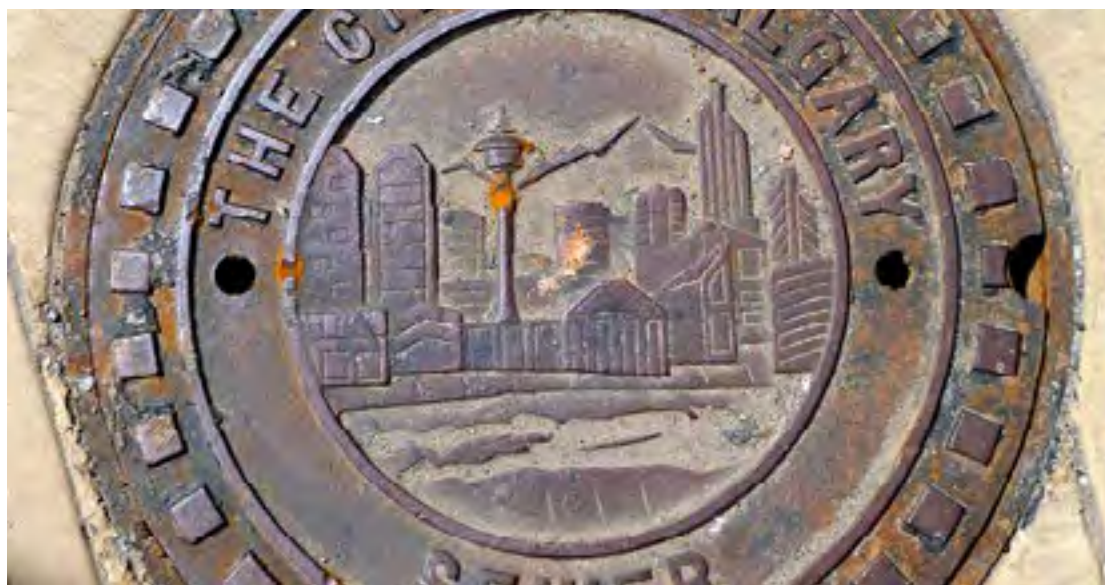
CATCH BASINS AND MANHOLE COVERS
