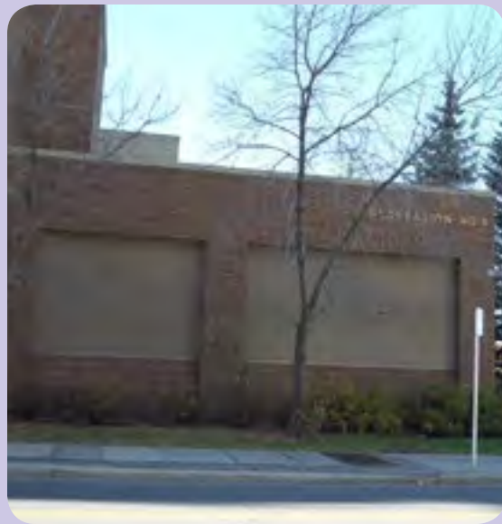
ENMAX BUILDING @ 8TH ST & 4TH AVE
