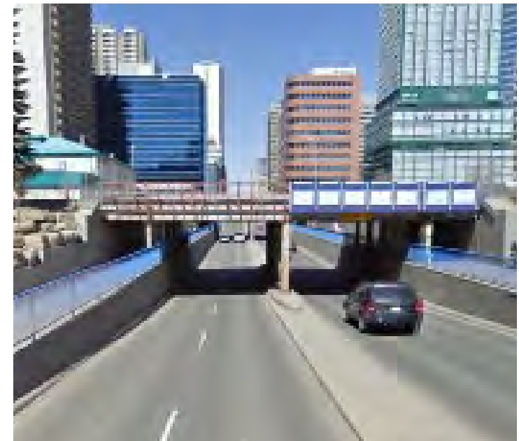
02 CPR BRIDGE - 8TH STREET
