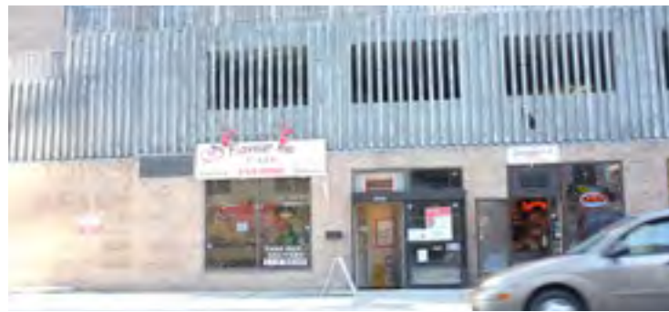
02 POOR COMMERCIAL FRONTAGE AND SOLID FACADES.
