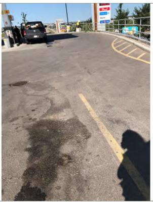
**Photo 25** Pavement staining leading to a drainage grate on the Shell gas station property on the southern side of CHB; adjacent the 14 Street NE and CHB intersection.
