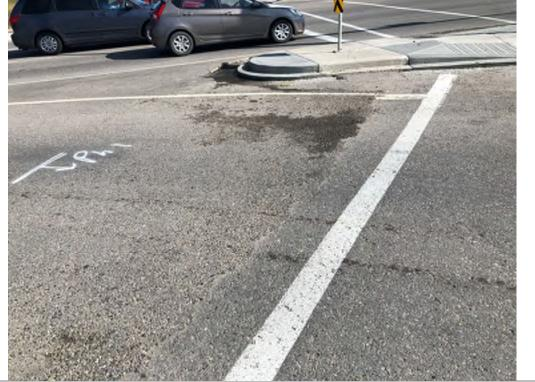
Photo 24 Pavement staining at the 14 Street NE and CHB intersection.
