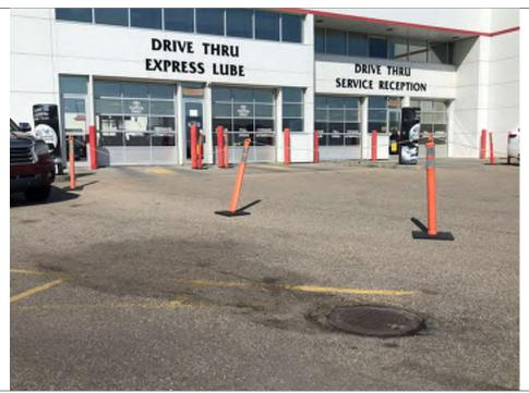
Photo 35 Pavement staining leading to a paved drainage area on the Country Hills Toyota dealership property.
