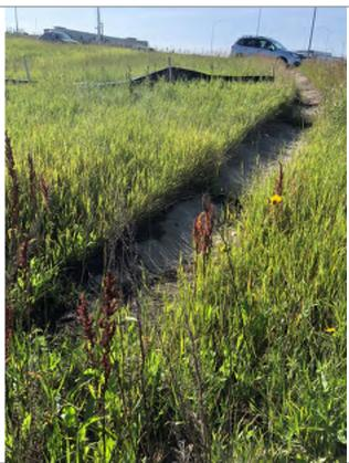
Photo 16 Stormwater drainage pathway for the northern side of CHB, leads to stormwater outfall "N<u>42"</u>.
