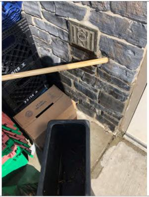
**Photo 29** Shell gas station up-close leaking water valve flowing out from the curve and onto their supplies.
