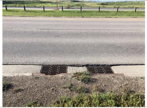
Photo 23 An example of the curbside paved drainage grates and catch basins along CHB.
