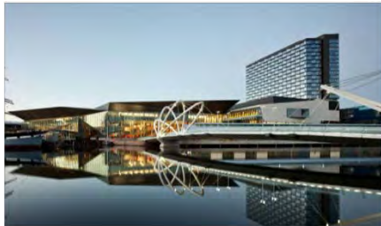
Melbourne Convention Center Melbourne, Australia
