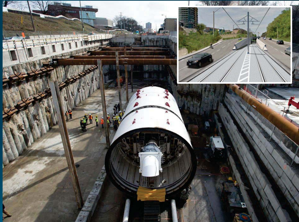
Eglinton LRT under construction, Toronto nationalpost.com
