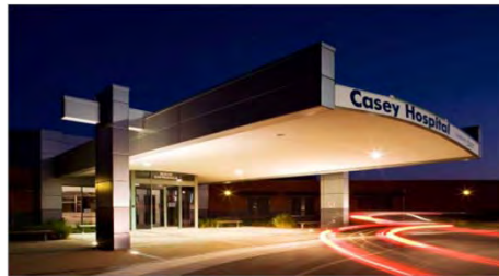
Casey Hospital Melbourne, Australia
