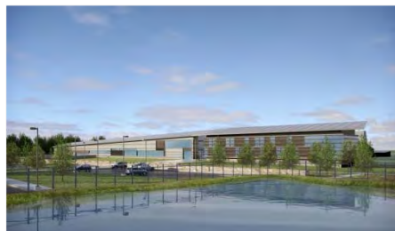
MGS New Data Centre Guelph, Ontario
