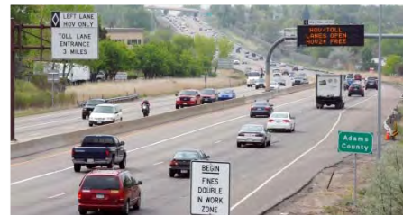
US 36 Concession Denver, Colorado
