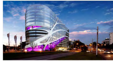
Victoria Comprehensive Cancer Centre Melbourne, Victoria, Australia
