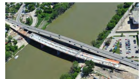
Disraeli Bridges Project Winnipeg, Manitoba
