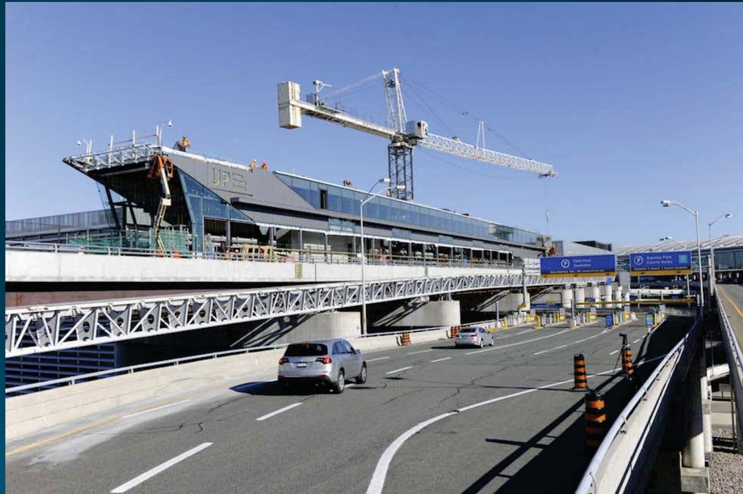
Union Pearson Express rail station under construction, Pearson International Airport transit.toronto.on.ca
