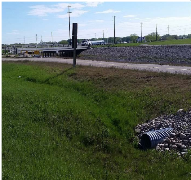
Figure 1.3: Southern canal culvert looking east
