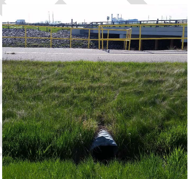
Figure 1.4: Northern canal culvert looking east
