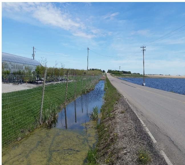
Figure 1.9: Western drainage ditch parallel to Road 284 looking north
