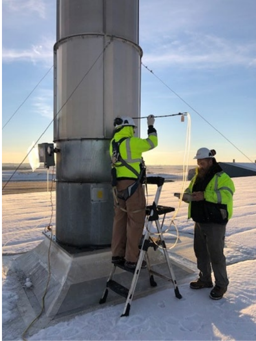
Photograph 5: Air sampling at a Biofilter Stack (flow measurements with Pilot tube and air sampling into Tedlar bag [at left of stack]) – looking northeast.
