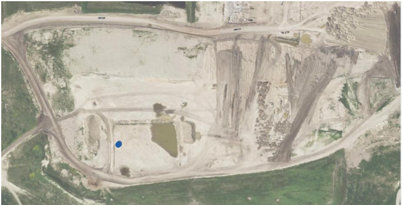
Figure 40. Aerial View of the Landfill Showing the Location of an Identified Surface Hotspot on the Landfill Cover
