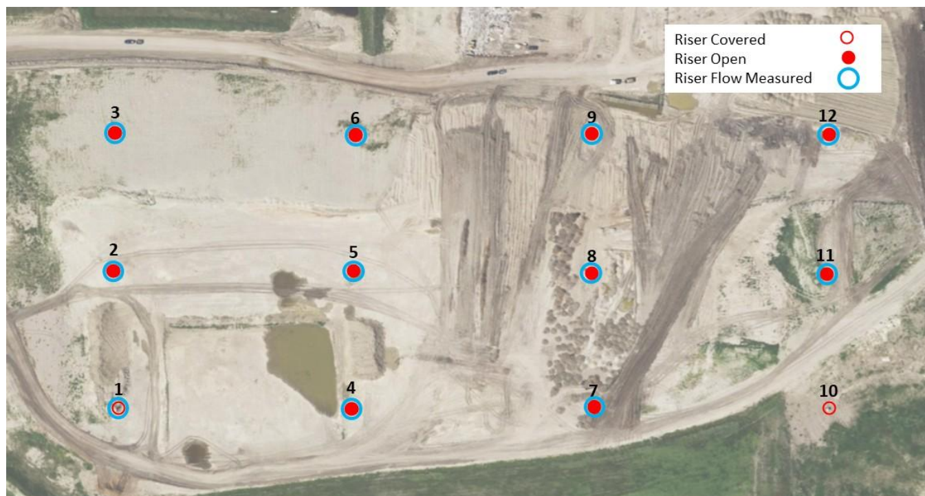
Figure 42. Aerial View of the Landfill Showing Riser Locations Confirmed as Important Sources of CH 4 and Odour
