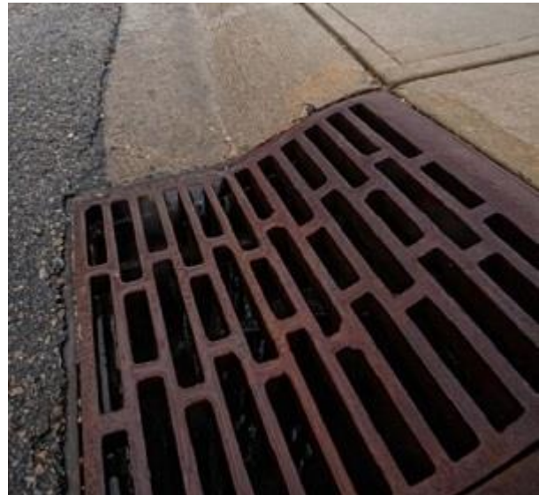
THE CITY OF CALGARY’S COMMUNITY DRAINAGE IMPROVEMENTS PROGRAM INVESTS IN UPGRADING THE STOMRWATER SYSTEM IN OLDER COMMUNITIES TO REDUCE THEIR SOTRMWATER FLOOD RISK.
