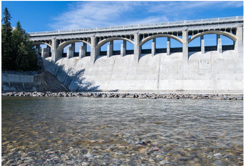
THE NEW UPGRADED GATES AT THE GLENMORE DAM REDUCE CALGARY’S FLOOD RISK ON THE ELBOW RIVER.
