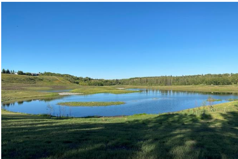
THE BEBO GROVE WET POND WILL ALLOW FOR STORAGE OF STORMWATER DURING RAIN EVENTS AND IMPROVE THE QUALITY OF THE WATER DISCHARGED TO FISH CREEK.
