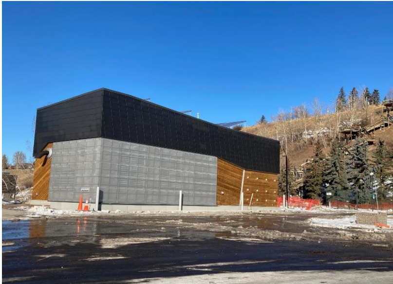
SUNNYSIDE PUMPSTATION #1 WAS COMPLETED IN 2020 WITH FUNDING SUPPORT FROM THE ALBERTA COMMUNITY RESILIENCE PROGRAM AND THE NEW BUILDING CANADA FUND TO REDUCE STORMWATER FLOODING IN THE COMMUNITY OF SUNNYSIDE
