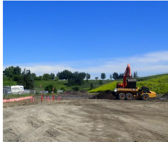
Site clearing, July 2020
