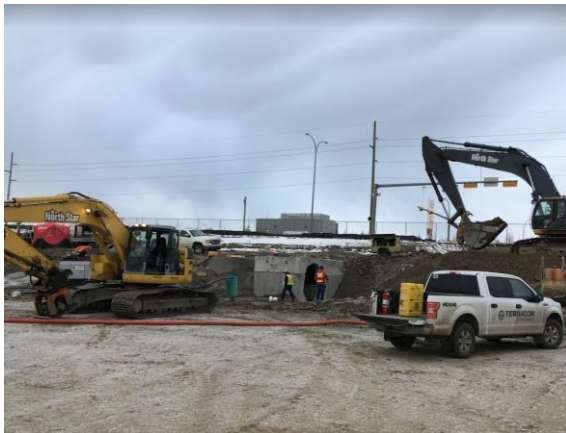
Crews installing underground utilities
