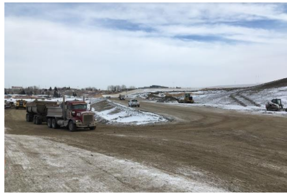
View of finished LRT embankment (right side of photo)
