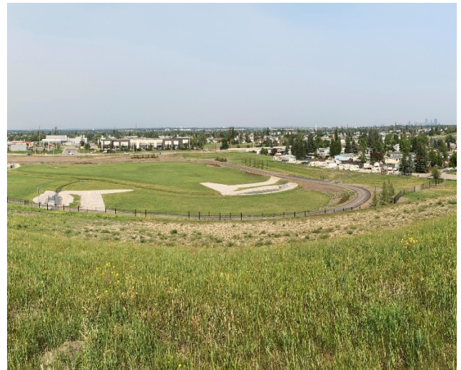
Looking west towards 24 St. SE – the new 'dry' storm pond and LRT embankment.
