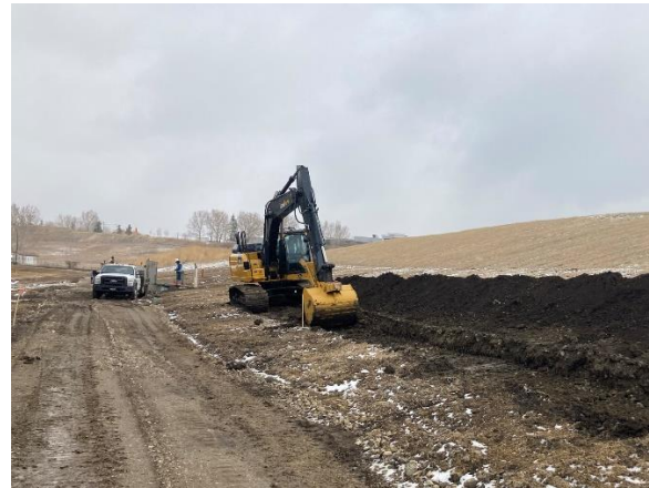
Landscaping Underway, April 2021
