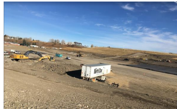
Installation of the pond underground structures
