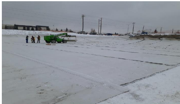
Working on the pond floor in sub-zero conditions
