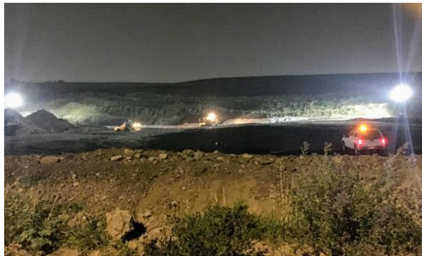
Working at night, September 2020
