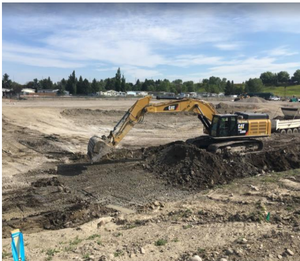
Removal of contaminated soil, August 2020
