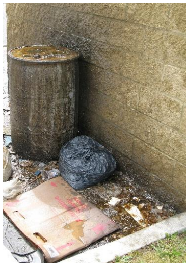
Figure 10 – Example of a poorly maintained used cooking oil barrel overflowing at the top, resulting in a FOG release.
