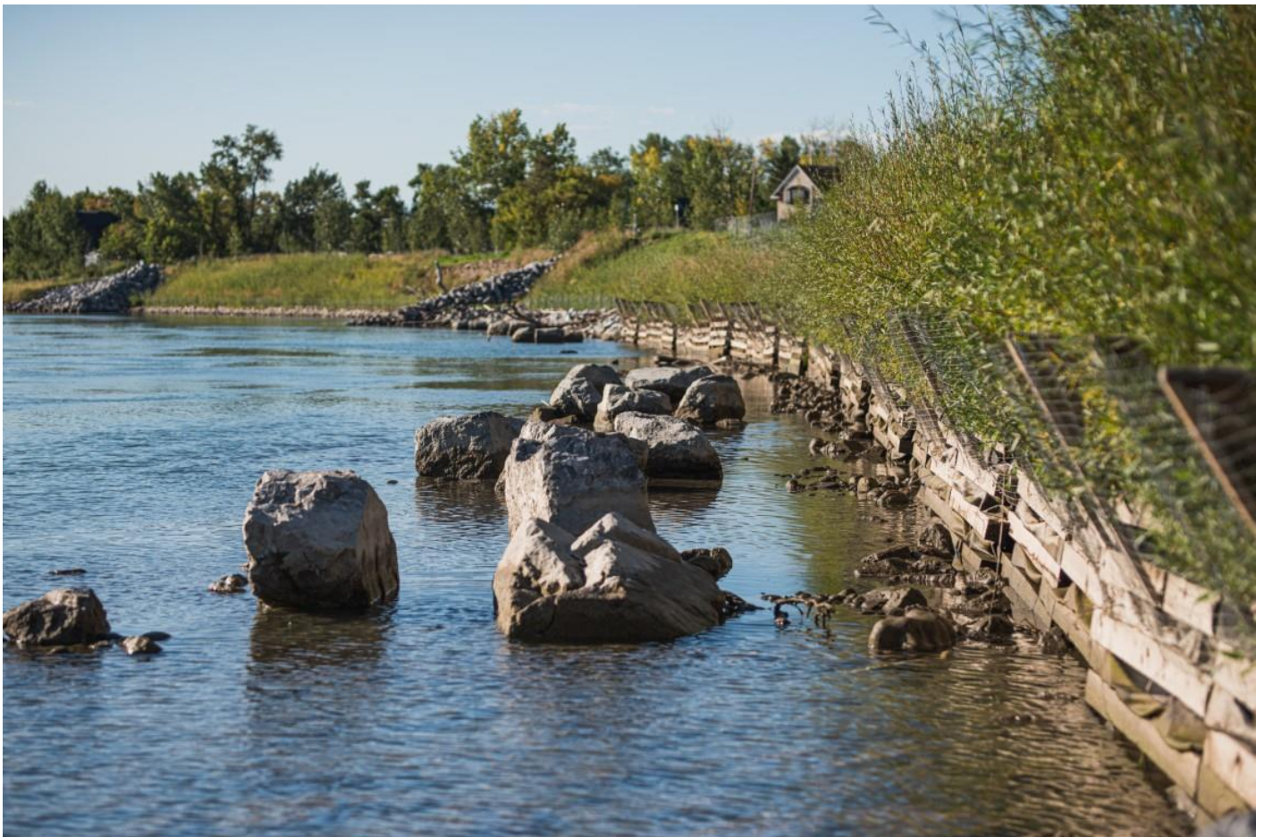
Photo 2-1: Timber crib wall and fish habitat enhancement boulders at Site 1-3.
