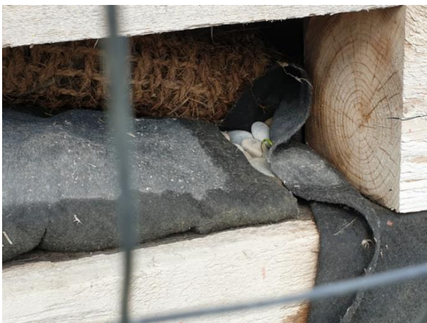
Photo 5-1: Gaps in non-woven geotextile used for material containment in the timber crib wall at Site 1-3
