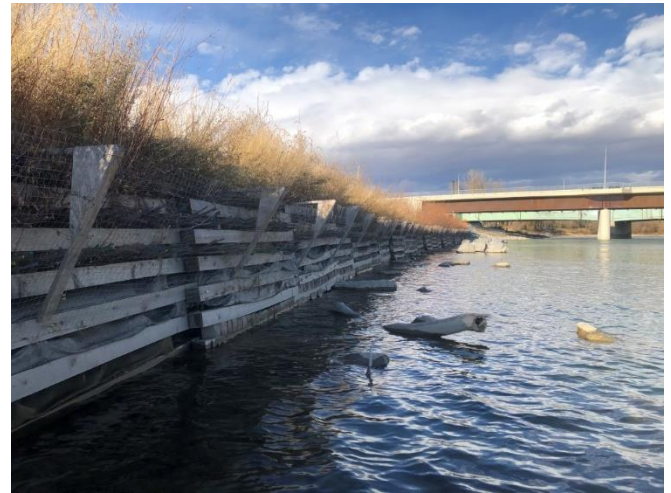
Photo 5-6: Fish shelters, fish habitat boulders and large woody debris (rodent protection fencing attached to face of crib wall) (October 25, 2019)
