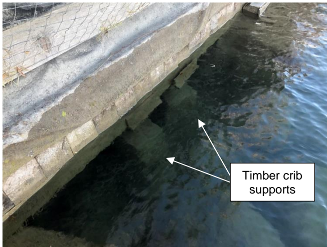
Photo 5-5: Fish shelter and timber crib supports (October 25, 2019)
