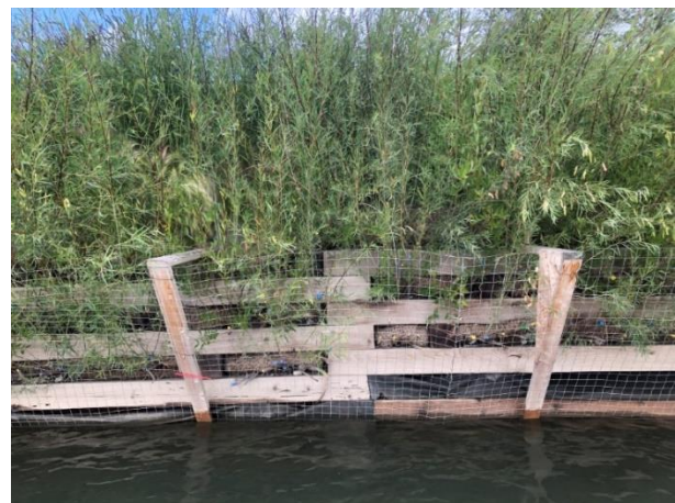
Photo 5-2: Typical vegetated timber crib wall section (shown with rodent fencing attached) (July 18, 2019)
