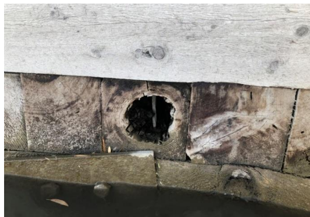
Photo 5-4: Crib wall timber with signs of dry rot (October 25, 2019)
