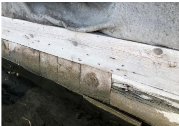
Photo 5-3: Crib wall timber with signs of insect damage and dry rot (October 25, 2019)
