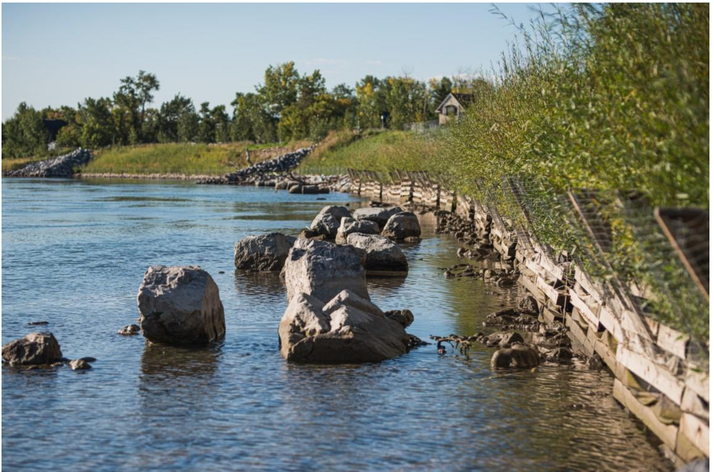
Photo 7-1: Timber crib wall and fish habitat enhancement boulders at BDEP.
