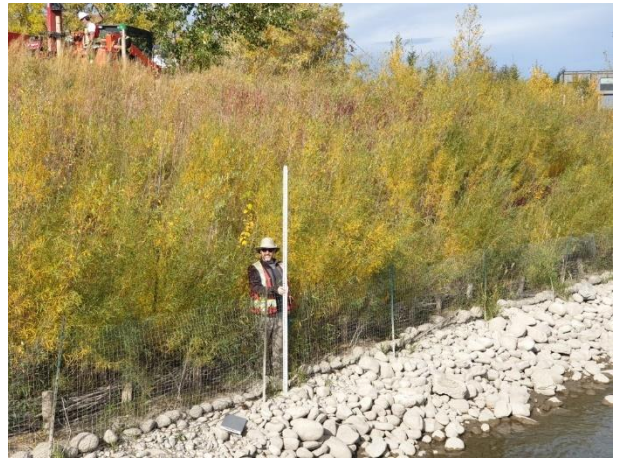
Photo 5-12: Good and vigorous growth in Hedge Brush Layer at Site 2 (September 25, 2020) Credit: Terra Erosion Control Ltd.
