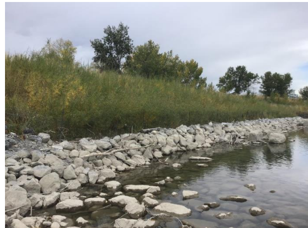
Photo E-16: Site 1 brush mattress with rock toe -note very good establishment (looking west)
