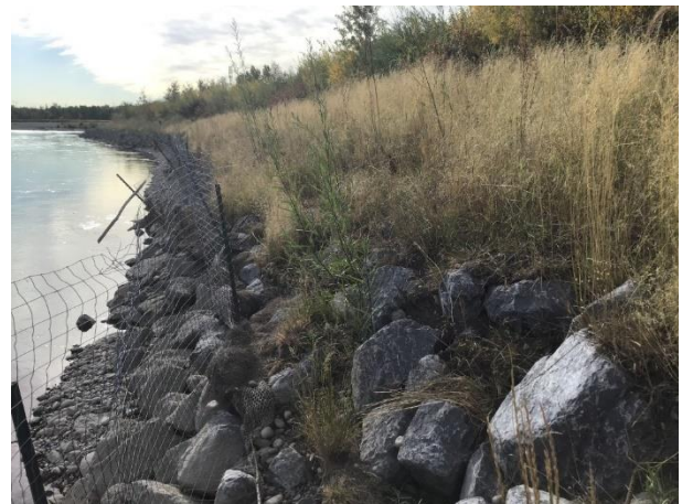
Photo 5-4: Degraded curlex log at Site 4 (Sept 25, 2020)
