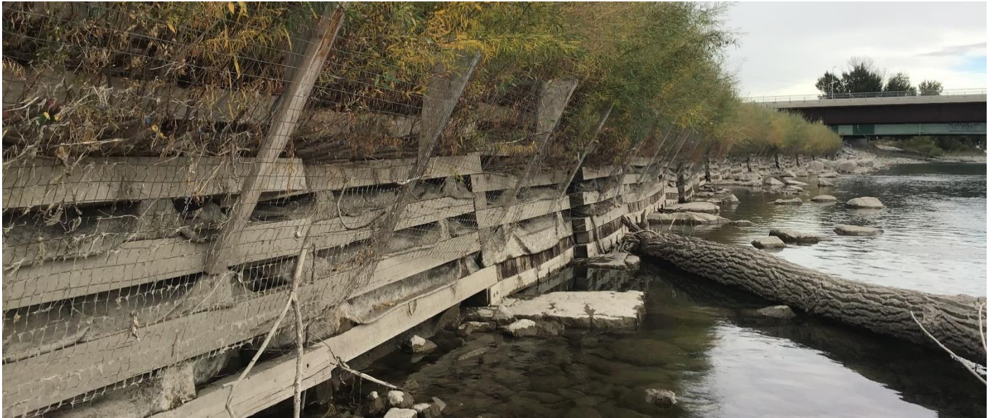
Photo 2-1: Timber crib wall and fish habitat enhancement boulders at Site 1-3.
