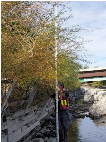
Photo E-19: Site 1 overhanging cover at vegetated timber crib wall (looking upstream)
