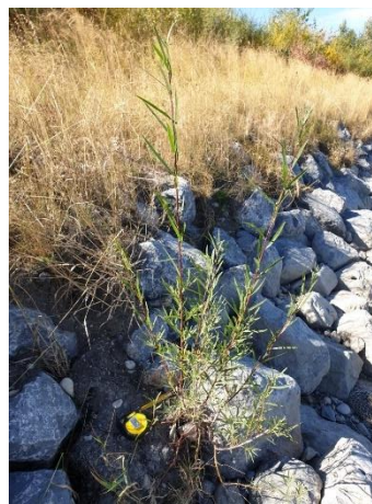
Photo 5-14: Live cutting at Site 4 (September 24, 2020) Credit: Terra Erosion Control Ltd.
