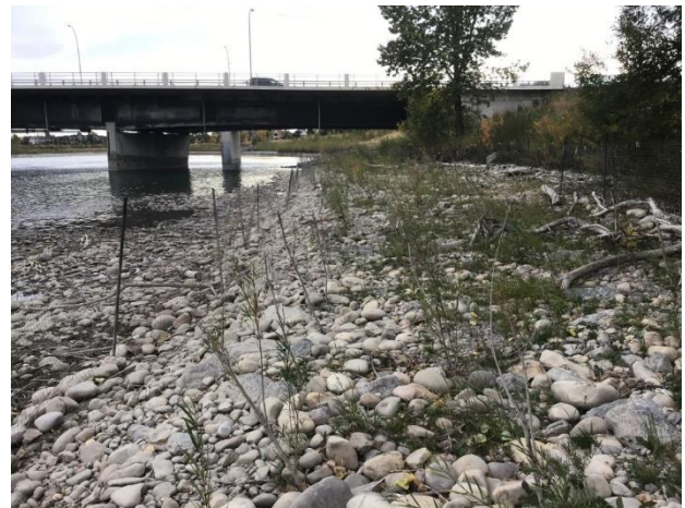
Photo E-4: Site 1 vegetated riprap with rooted live cuttings wildlife corridor upstream of Cushing bridge (looking downstream)
