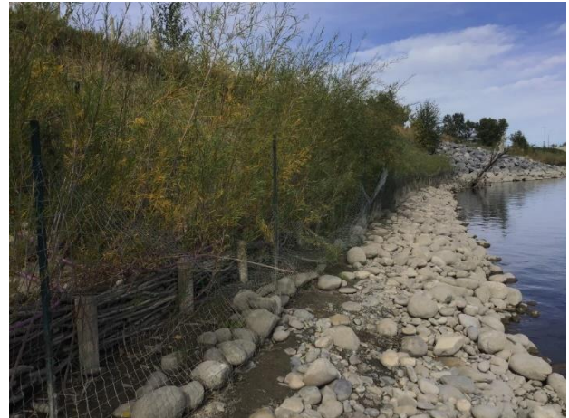
Photo E-26: Site 2 box fascine toe –no toe erosion observed (looking upstream)
