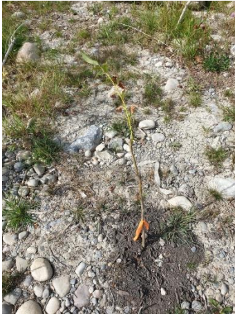
Photo E-17: Site 1 replanted live cuttings in vegetated riprap upstream of Cushing Bridge
