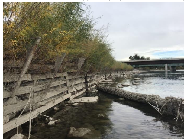
Photo 5-8: Timber crib wall at Site 1
