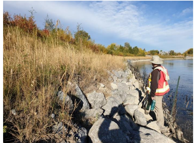
Photo E-38: Site 4 – note erosion of placed toe fill material – observed to be no further erosion in 2020 (looking upstream)
