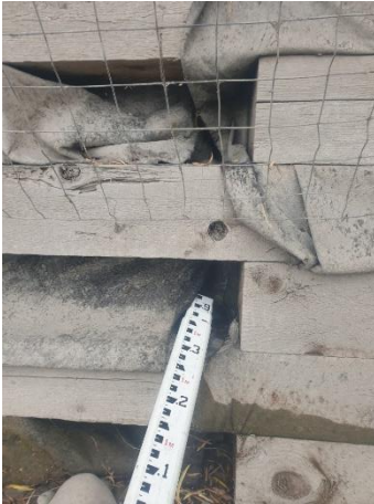
Photo E-13: Site 1 gap in containment materials in the vegetated timber crib wall
