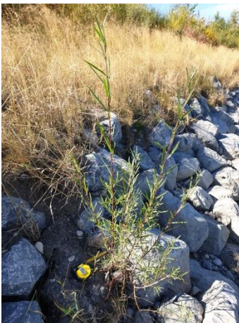
Photo E-43: Site 4 live cutting established around riprap (looking upstream)
