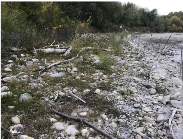
Photo E-3: Site 1 vegetated riprap with rooted live cuttings wildlife corridor upstream of Cushing bridge (looking upstream)
