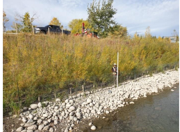
Photo E-30: Site 2 hedge brush layer establishment and no toe erosion observed
