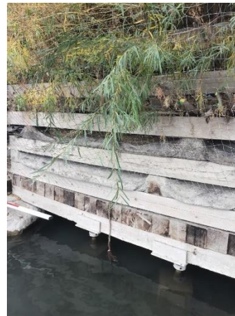
Photo E-8: Site 1 Vegetated timber crib wall – willow roots extending down into the river
