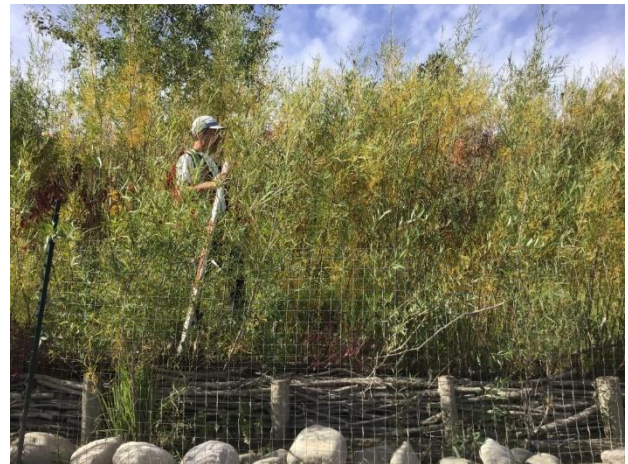
Photo E-28: Site 2 hedge brush layer and box fascine with good establishment (looking west)
