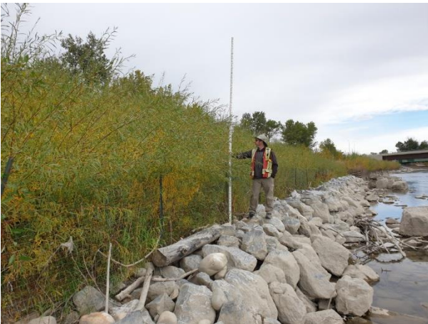
Photo E-15: Site 1 brush mattress with rock toe -note very good establishment (looking upstream)
