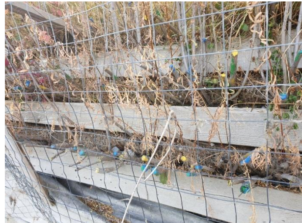
Photo E-20: Site 1 dead cuttings in timber crib wall
