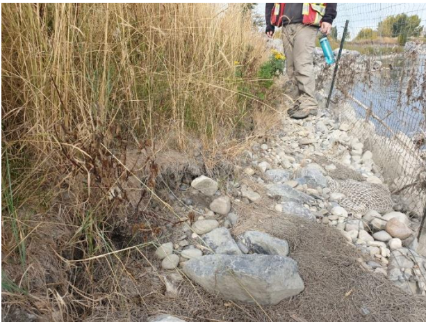
Photo E-39: Site 4 condition of curlex log (looking upstream)
