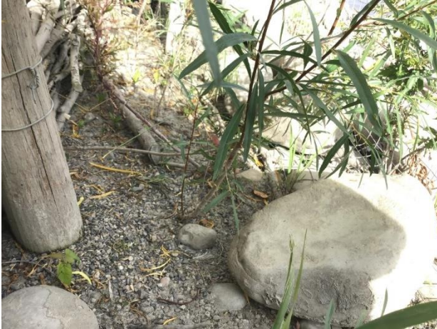
Photo E-29: Site 2 brush layer under box fascine establishment – also note good condition of wood posts and steel wire
