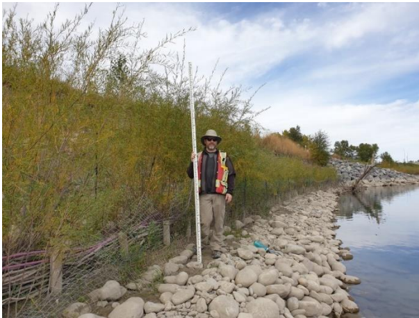
Photo 5-11: Box fascine growth at Site 2 (September 25, 2020) Credit: Terra Erosion Control Ltd.
