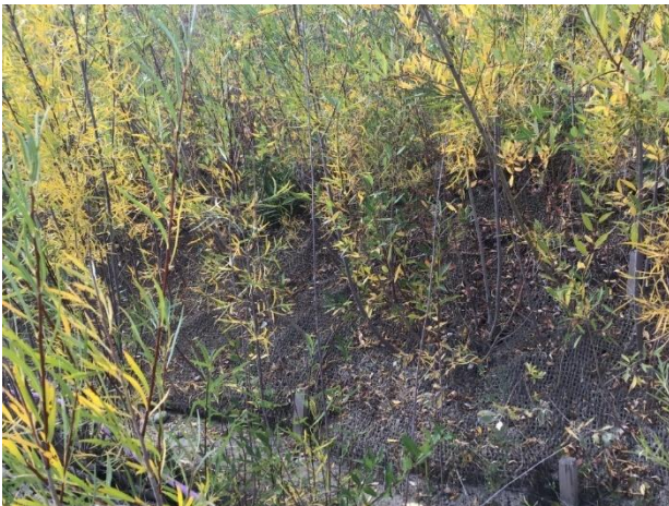
Photo E-27: Site 2 biodegradable coir geogrid in good condition
