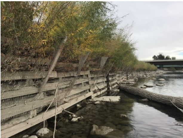
Photo E-7: Site 1 Vegetated timber crib wall (looking upstream)
