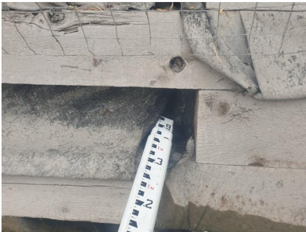
Photo 5-1: Gaps in non-woven geotextile used for material containment in the timber crib wall at Site 1 Credit: Terra Erosion Control Ltd.
