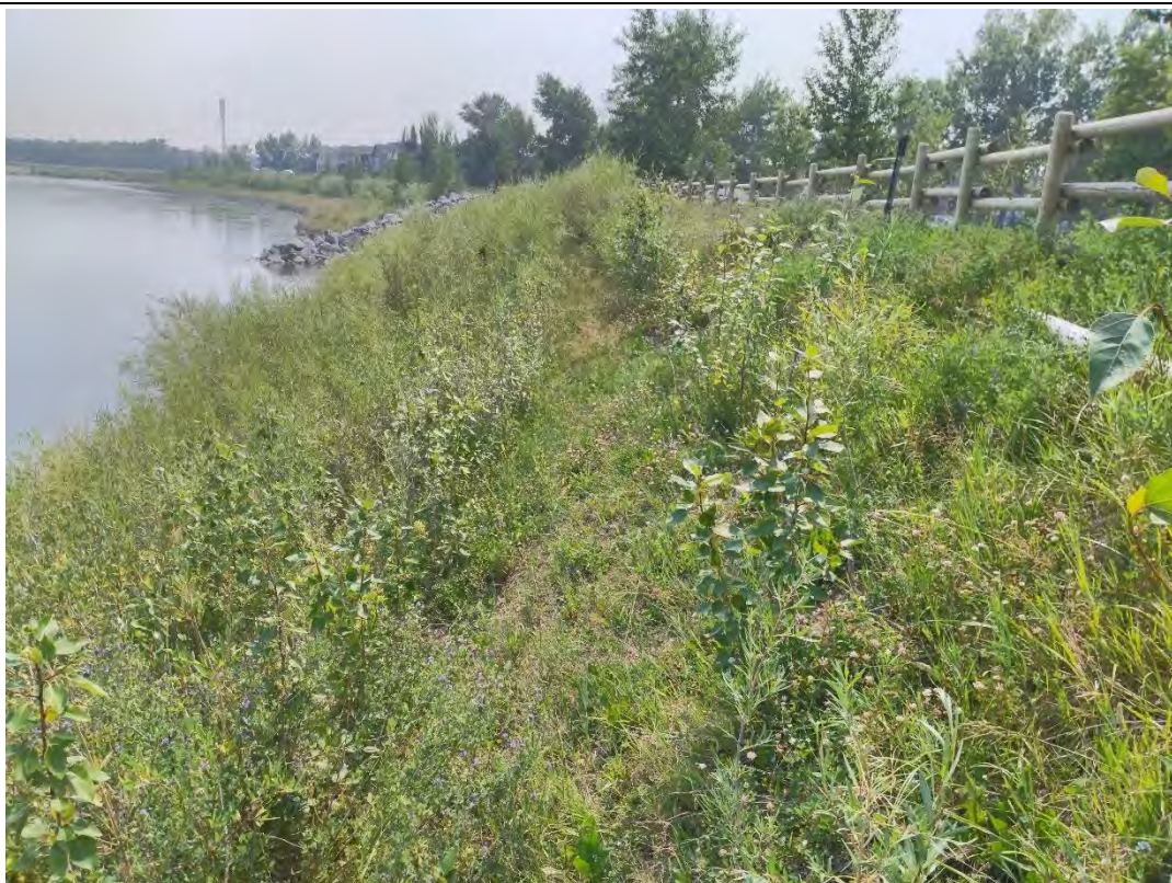
RHIP95BOW056 (2021, Waypoint 2C) – View downstream in Site 2 – successful implementation of box fascine with brush layering and slope treatment. Wood rail fencing at the top of the bank should be retained to curtail recreational access to bank bioengineering treatments in the long-term. (Photographer: K. Hull)
