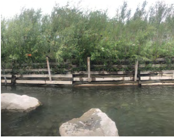
Photo 5-2: Timber crib wall, rock riprap (submerged), and fish boulders (July 21, 2021).
