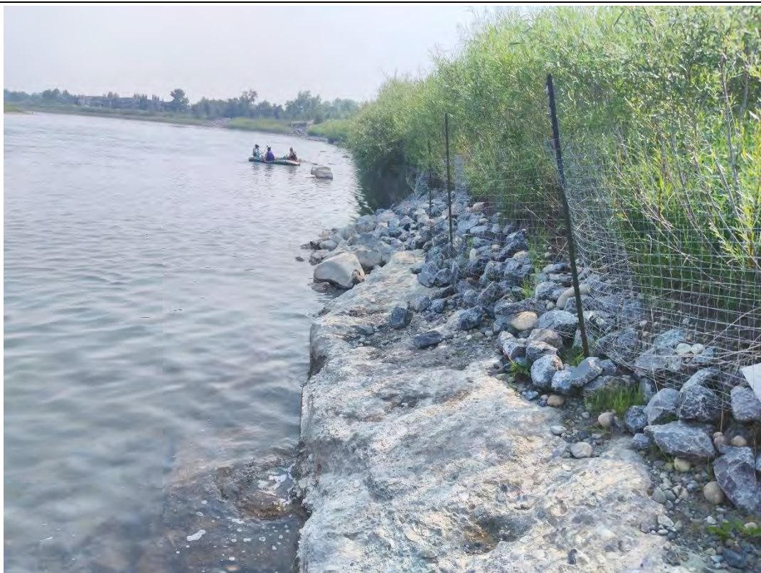
RHIP95BOW071 (2021, Waypoint 2H) – View downstream at the upper end of Site 1-3 – showing excellent establishment of sandbar willows within the timber crib wall. Fencing in the foreground at the base of the bank has been built to exclude beaver access. (Photographer: K. Hull)
