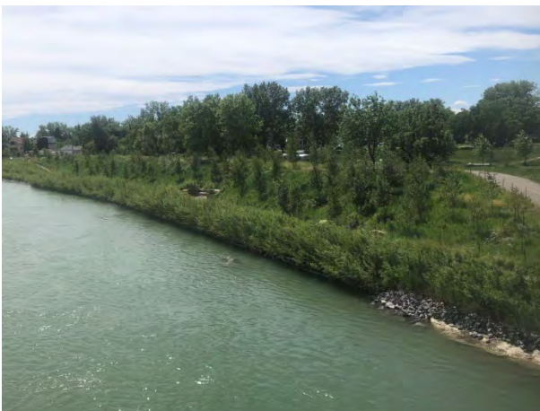
Photo 5-12: Good and vigorous growth at timber crib wall, vegetated soil wraps and riparian area of Site 1 – looking downstream (June 18, 2021)
