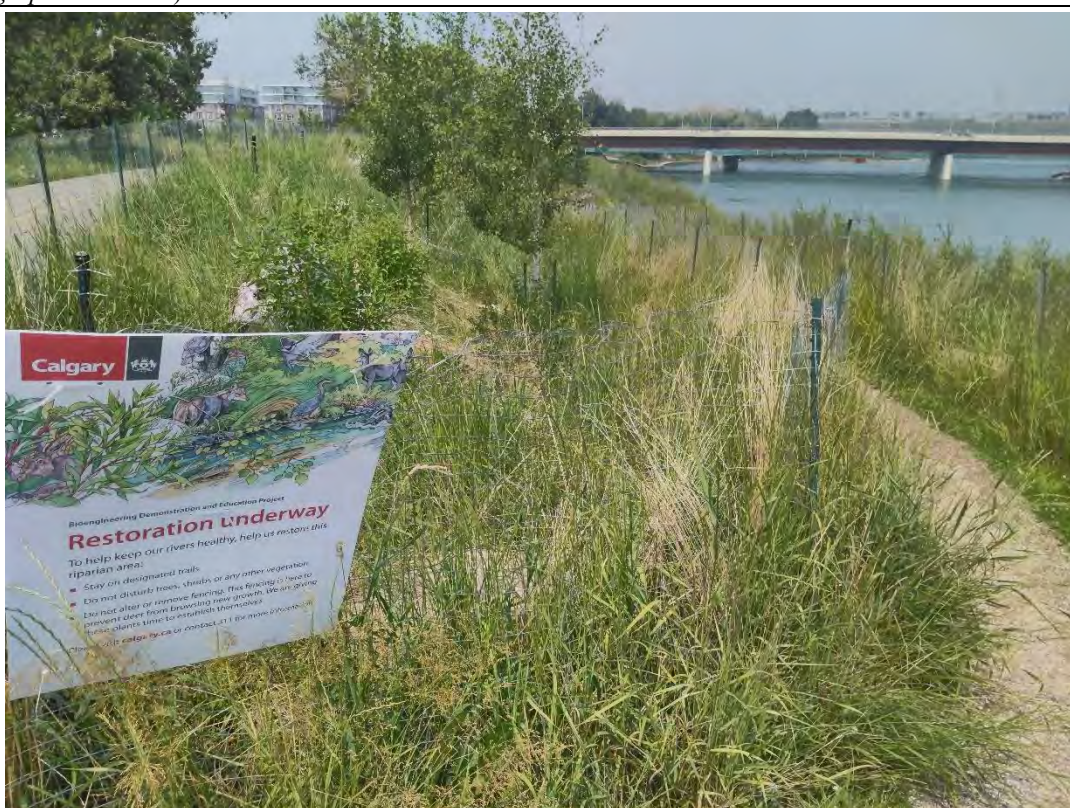
RHIP95BOW063 (2021, Waypoint I) – View upstream to the Cushing and BRT bridges from the lower end of Site 1-4. This portion of bank was reshaped to accommodate a wildlife corridor and lower riparian terrace. Dense cover from seeded grasses may be limiting to riparian plantings here. (Photographer: K. Hull)
