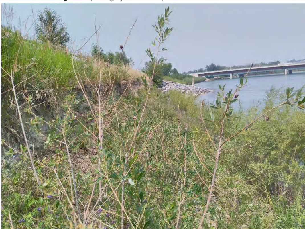
RHIP95BOW057 (2021, Waypoint 2C) – View upstream within Site 2 – successful box fascine at the toe, no slope treatment above due to steep exposed cutbank with swallow nests. (Photographer: K. Hull)
