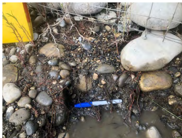
Photo 5-17: Root growth into native substrates at the toe of Site 2 (July 20, 2021)
