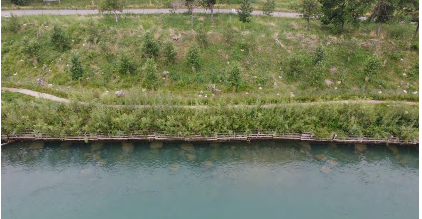
Photo 2-1: BDEP timber crib wall, fish shelters and habitat enhancement rocks at Site 1 (July 21, 2021)
