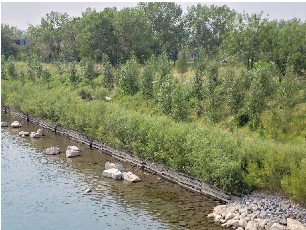
MONT95BOW0005 (2021) – View upstream from the BRT bridge viewing platform showing Site 1-3 , timber crib wall. Excellent establishment of native plantings have augmented root mass protection, enhanced overall woody cover and wildlife habitat structure. (Photographer: K. Boehler)
