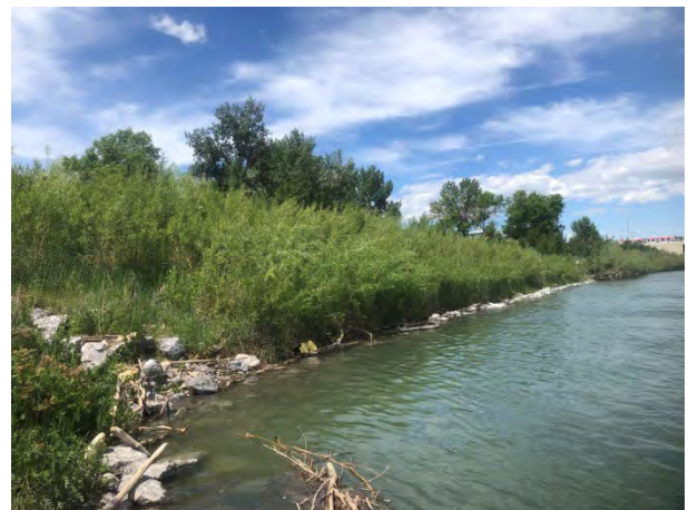
Photo 5-13: Good and vigorous growth in brush layers and brush mattress at downstream end of Site 1 – looking upstream (June 18, 2021)
