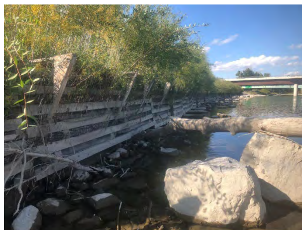
Photo 5-9: Timber crib wall at Site 1 on September 13, 2021
