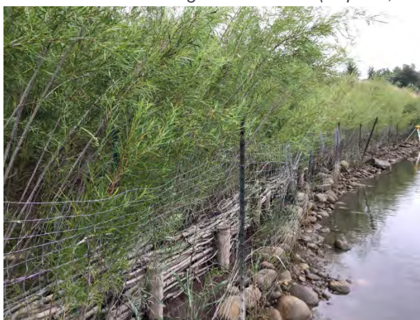
Photo 5-8: Temporary rodent fencing at Site 2 (July 20, 2021)
