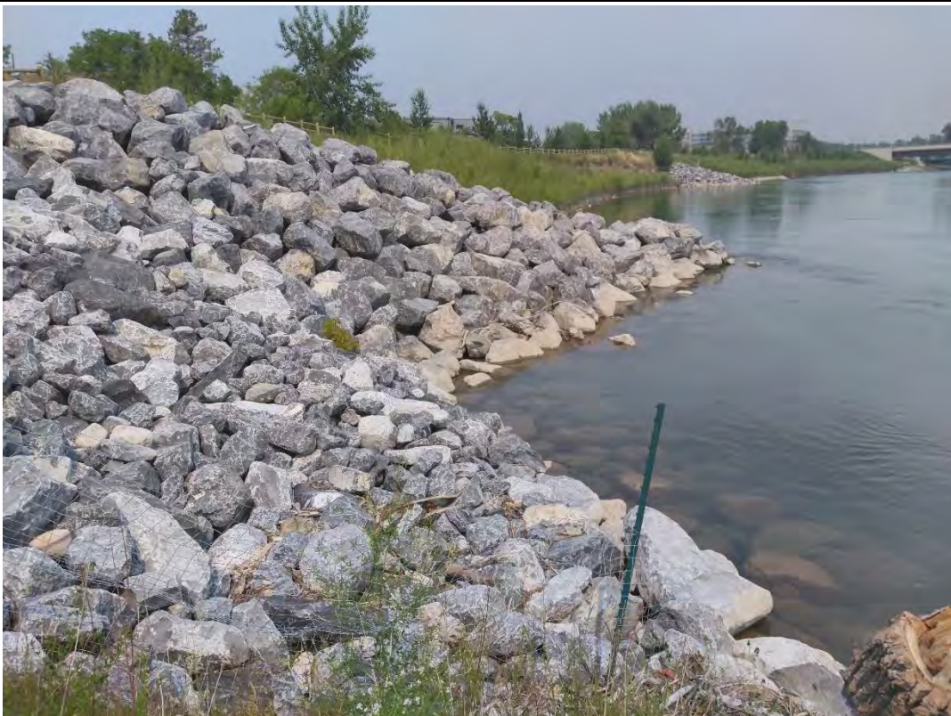
RHIP95BOW047 (2021, Waypoint 2A) – In addition to unvegetated riprap at the downstream end, two large riprap rock groynes were unmodified since 2016. Structural alterations like these detract from the riparian health score. (Photographer: K. Hull)
