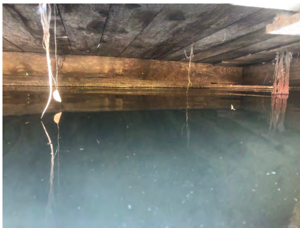
Photo 5-6: View under the fish shelter structure in the timber crib wall. Note the roots growing through the structure and extending into the water (Sept 13, 2021)
