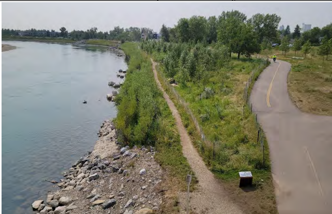
MONT95BOW0002 (2021) – View upstream from the BRT bridge viewing platform showing the BDEP site and successfully established plantings in addition to the reshaped bank and wildlife corridor and repositioned regional paved pathway. (Photographer: K. Boehler)
