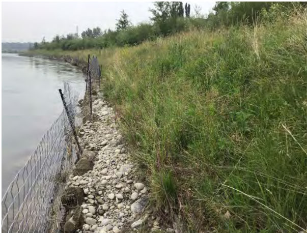
Photo 5-4: Degraded Curlex® Sediment Log® and temporary rodent fence at Site 4 (July 19, 2021)
