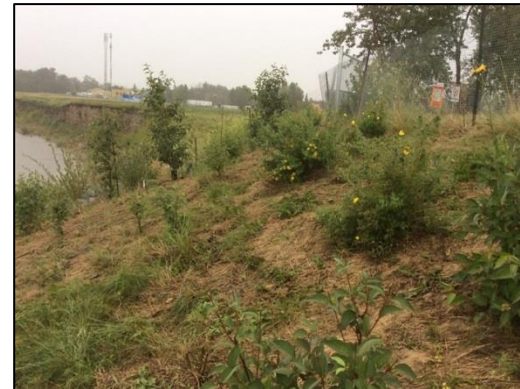
Photo 4: Close-up of Site 4 post-flood bank reconstruction with riparian planting above riprap.
