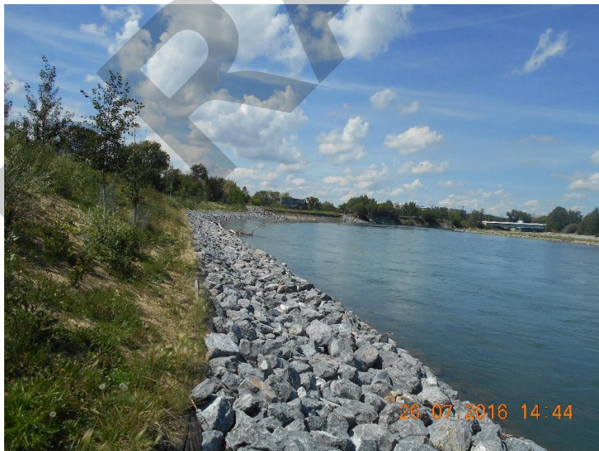
Photo 12. Looking northwest. Riprap along the river bank of Site 4.
