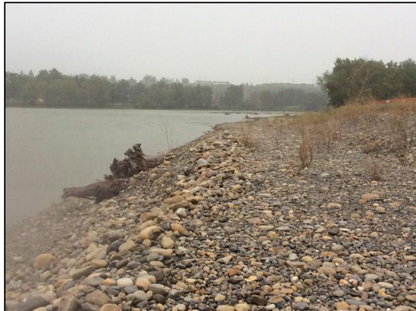
Photo 7: View taken from constructed gravel bar. Gravel re-located from Site 3 during post-flood reclamation activities.
