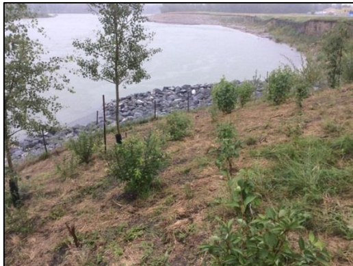
Photo 3: Site 4 post-flood bank reconstruction with riparian planting above riprap.
