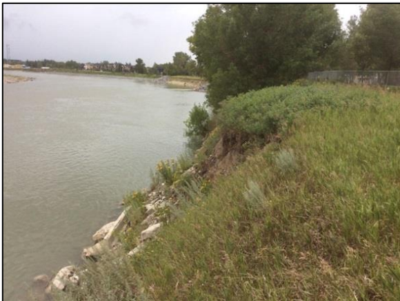
Photo 3: View looking downstream from middle of Site 1. View of historic broken concrete remediation and steep slope.
