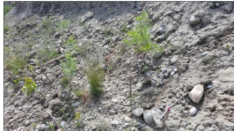
Photo 4: View of historic live staking in eroded bank.
