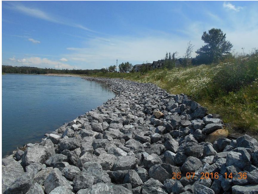
Photo 11. Looking southeast. Riprap along the river bank of Site 4.
