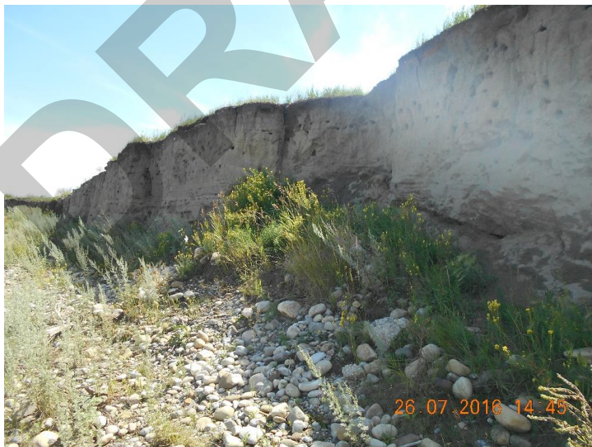
Photo 14. Looking south. Erosion near top of bank of Site 5 and exposed soil stratigraphy.
