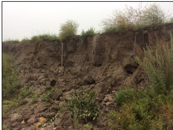
Photo 3: Close-up of overflow from swale from riparian bench above.
