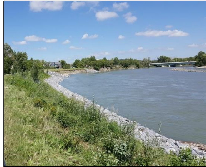
Photo 6: Looking upstream at Site 4 rip rap and riparian planted area from top of bank.
