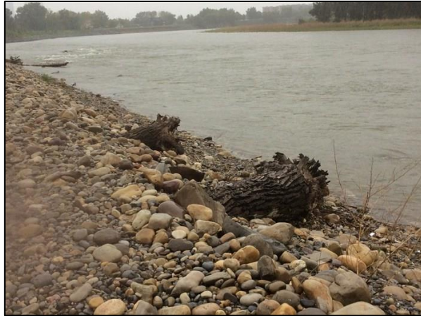
Photo 5: View taken from constructed gravel bar on Site 5 noting large woody debris buried as part of previous post-flood reclamation activities.
