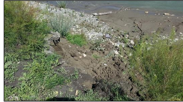
Photo 10: Post rainfall runoff deposition of eroded sediments via swales constructed in the re-contoured and reclaimed riparian bench.
