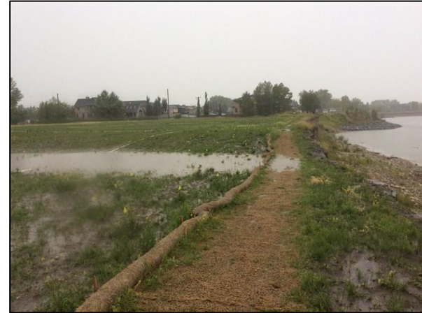
Photo 2: Note runoff through swale on riparian bench flowing toward river.
