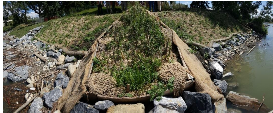
Photo 7: July 18, 2016. View of live groyne component above rip rap for the City of Calgary Bioengineering project.
