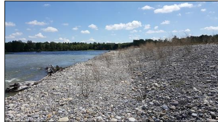
Photo 12: Dried and desiccated vegetation on constructed gravel bar placed from Site 3. Note the lower bench available for active mobilization.
