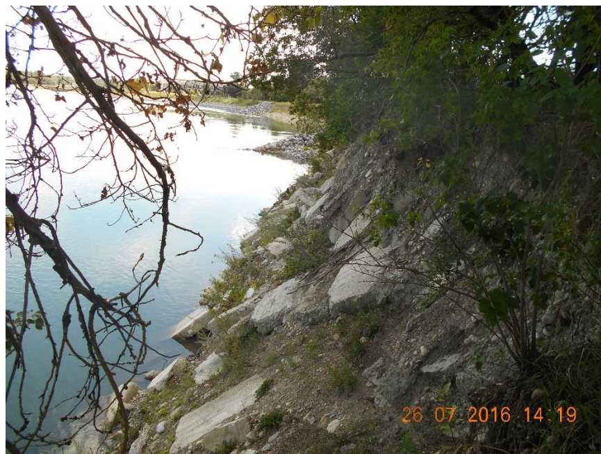
Photo 5. Looking south. Eroded river bank of Site 1 and concrete debris.
