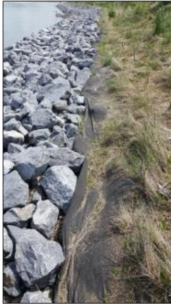
Photo 5: June 2, 2016 – Exposed filter material shows extent and use of synthetic materials in construction at transition from rip rap to riparian planting area.
