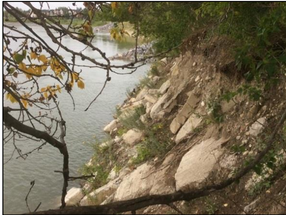
Photo 5: View at downstream end of Site 1. Steep slope with historic broken concrete remediation.
