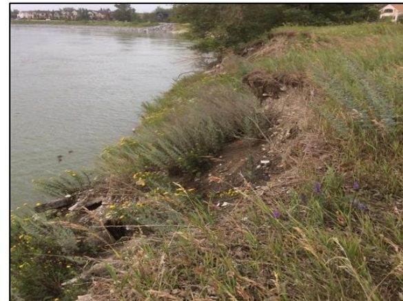
Photo 4: Looking towards downstream end of Site 1. Localized bank slump.
