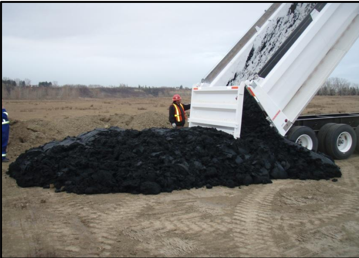
Photograph 5: Dewatered biosolids are transported using end-dump trailers and stockpiled at a marginal land reclamation project near
