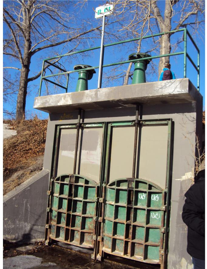
Figure 16 - Slide Gate Example
