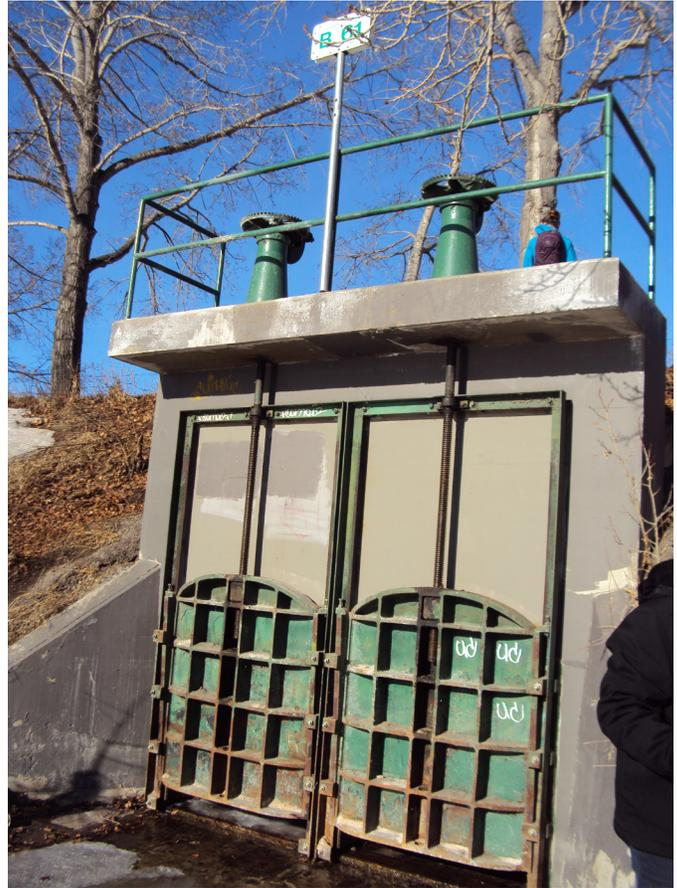
Figure 16 - Slide Gate Example
