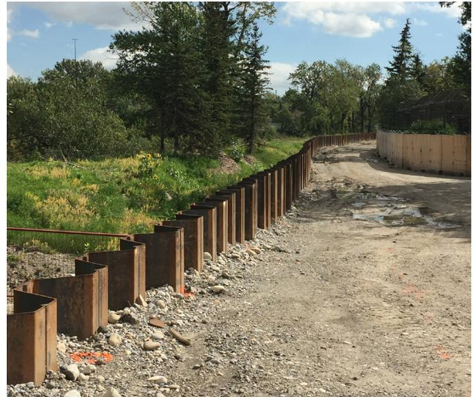
Figure 14 - Sheet Pile Wall Example
