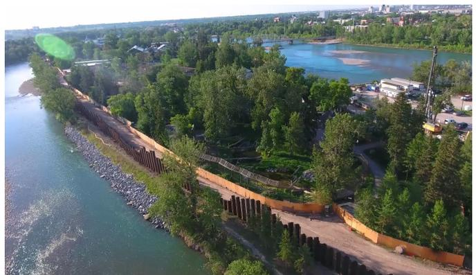
Figure 15 - Sheet Pile Wall Example
