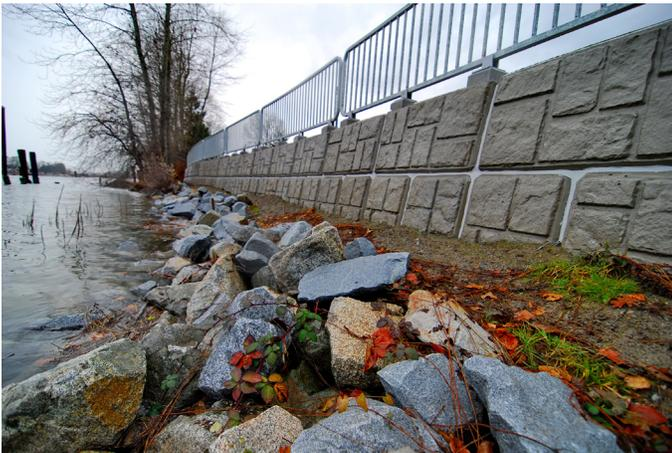
Figure 11 - Floodwall Example
