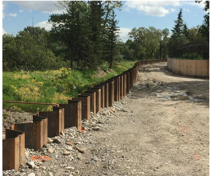
Figure 14 - Sheet Pile Wall Example
