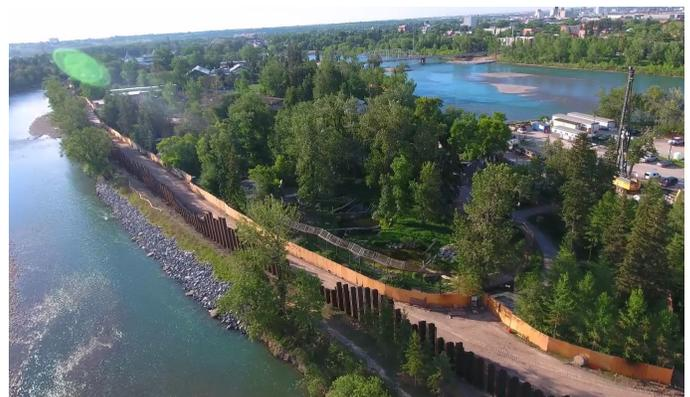
Figure 15 - Sheet Pile Wall Example
