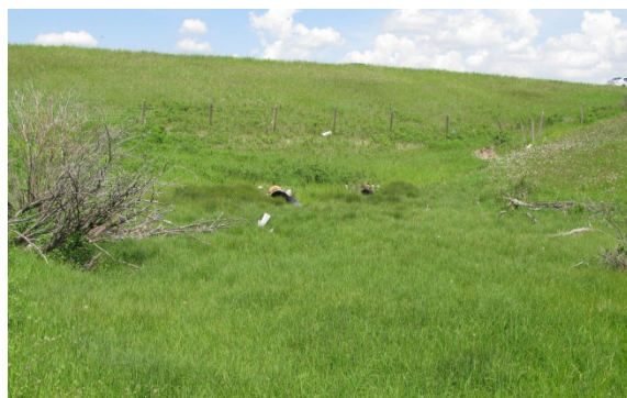
Photo 1 – South end of Coach Creek Culverts 'A' under Trans Canada Highway.
