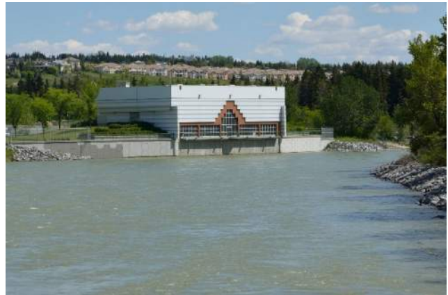
Photograph 1 Bearspaw WTP on north bank of the Bow River (courtesy Rick Carnduff).
