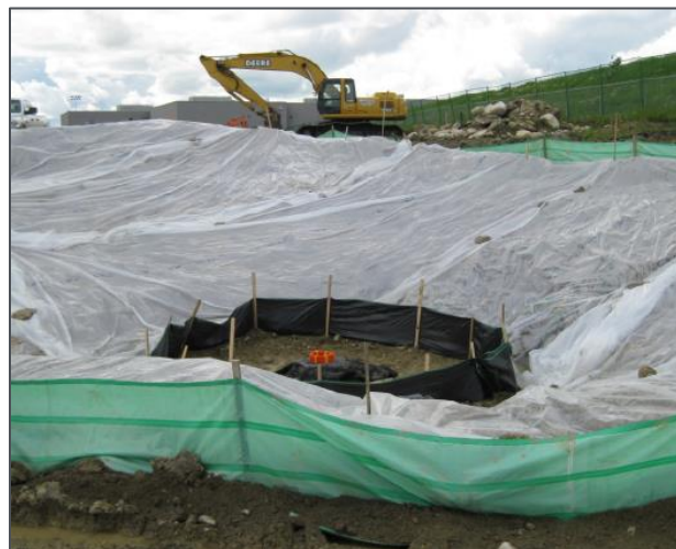
Photo 7 Isolation measures, poly sheeting
