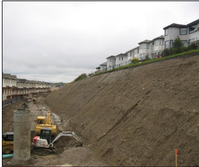
Photo 14 Steep slope created to facilitate infrastructure installation
