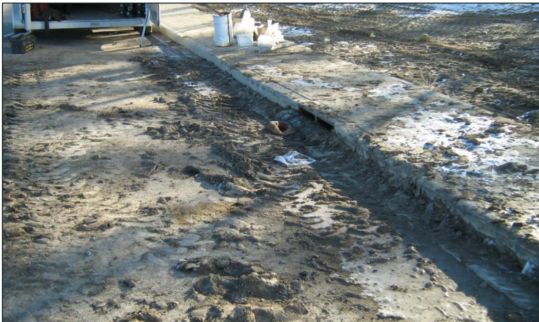
Photo 3 Mud tracked onto roadway and over a catch basin
