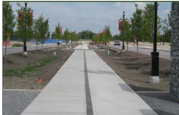
Photo 6 Installing low-impact developments last is the preferred construction method
