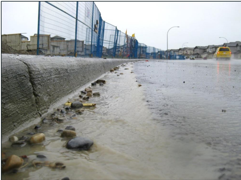
Photo 1 Sediment laden water flowing off a construction site
