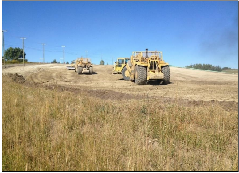
Photo 4 Stripping and grading using earth movers
