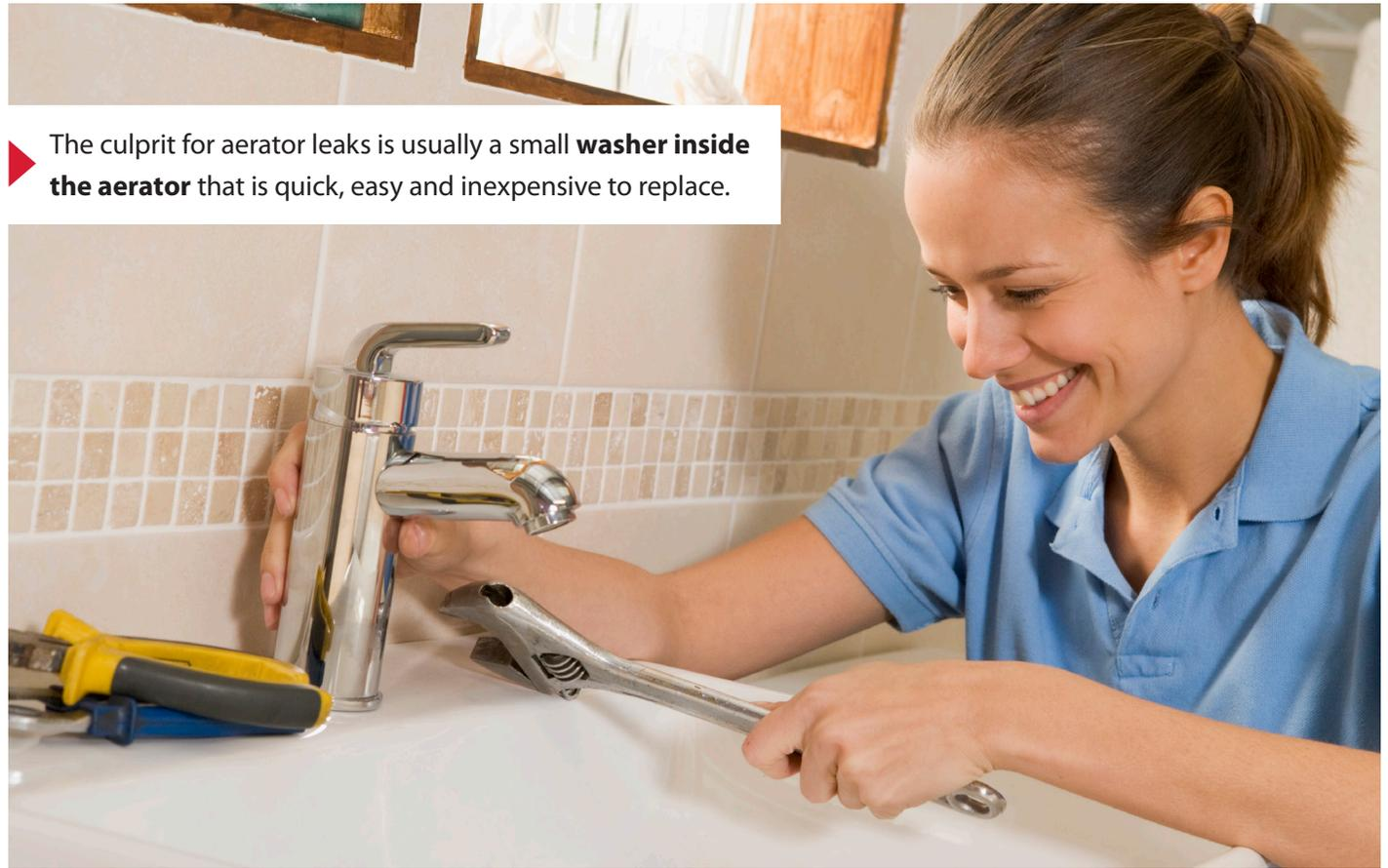
▶ The culprit for aerator leaks is usually a small **washer inside the aerator** that is quick, easy and inexpensive to replace.
