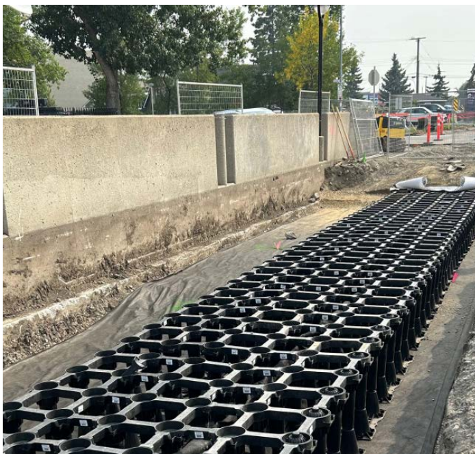
Soil cells being installed in Inglewood/Ramsay, which was supported by the Stormwater Redevelopment Fund.
