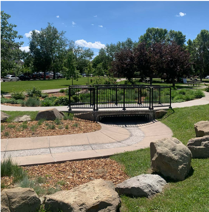
Riverside Park bioretention asset.
