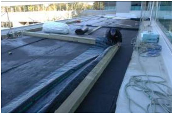
(e) Installation of root barrier
