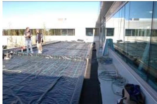
(f) Installation of Root Barrier
