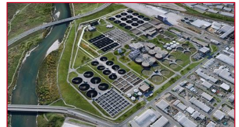
Bonnybrook Wastewater Treatment Facility
