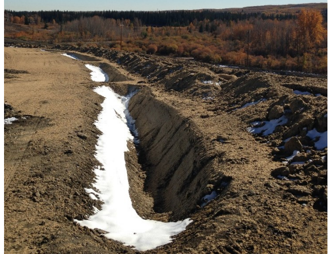
Photo 1: V-ditch with berms and mulch and tackifier cover
