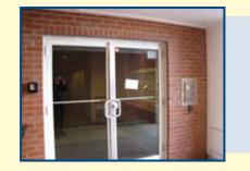
This entry is designed with an anti-jimmying plate on the door, an outside intercom, a security camera and glass security doors which provides the tenants with access control and good surveillance. This also increases security at the site and reduces fear for tenants.
