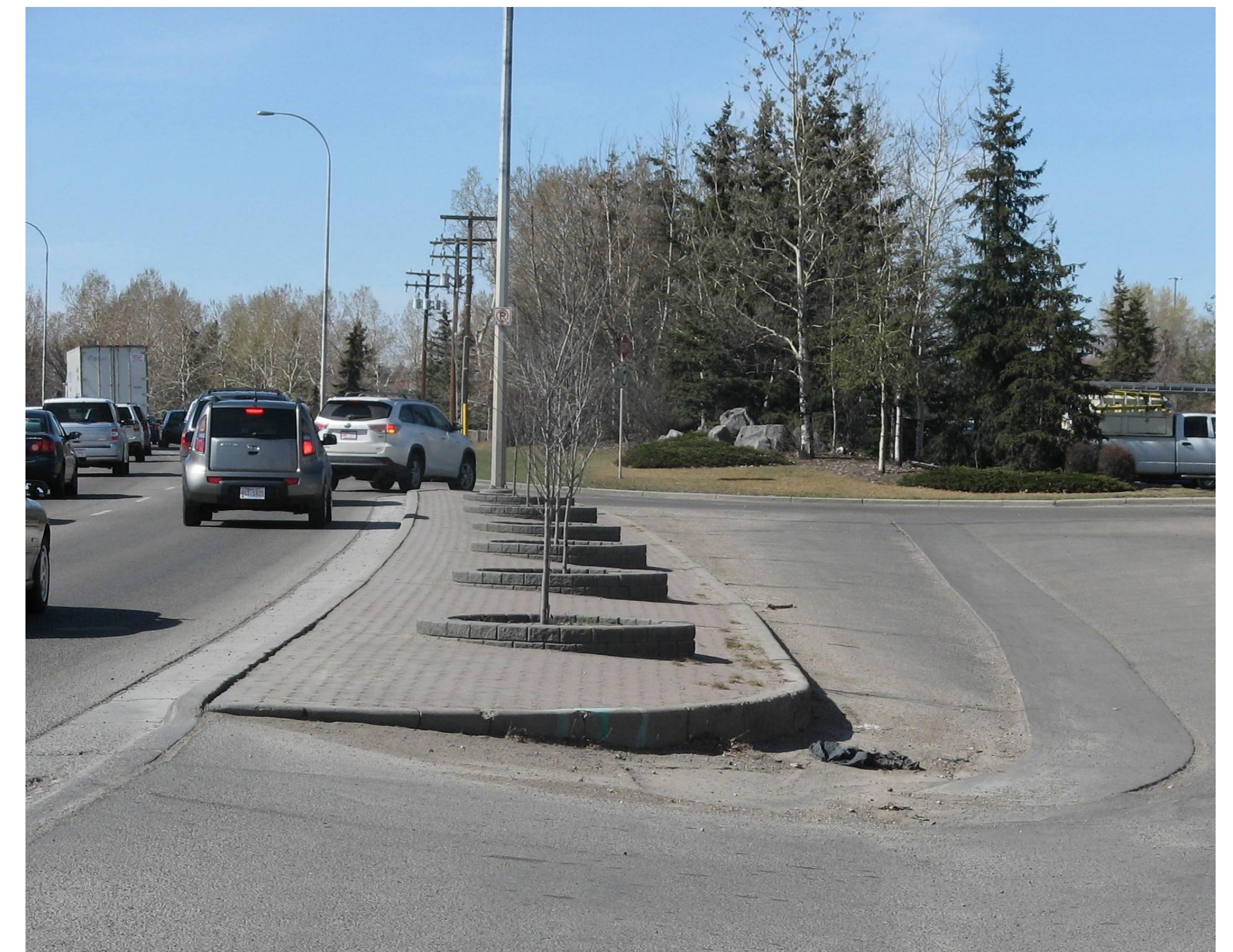
Westbound 16 Avenue N.W. just west of Home Road.
