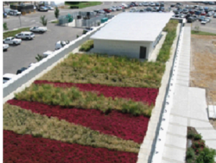
Figure 13 | Green roof The Water Centre, Calgary, AB
