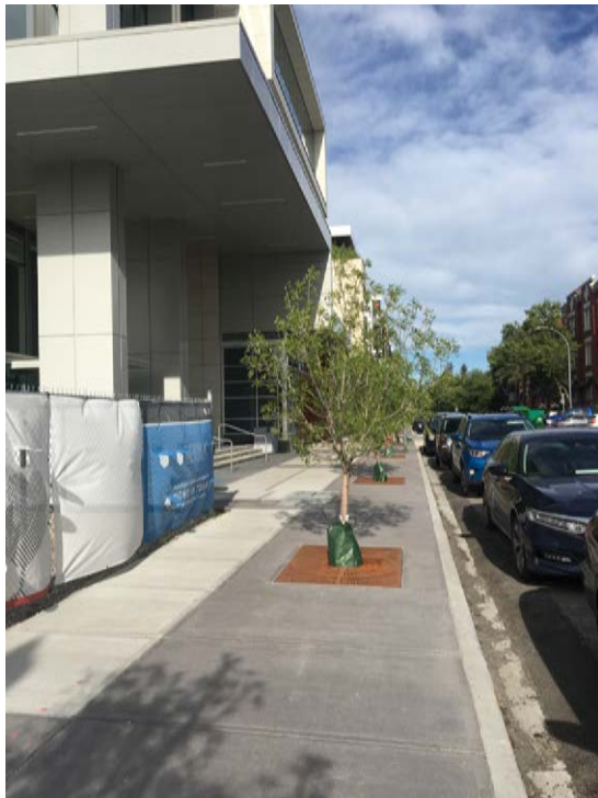
fig. 11 - sidewalk condition along 16th ave. sw
