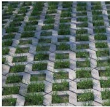
Site Drainage - Permeable Surfaces
